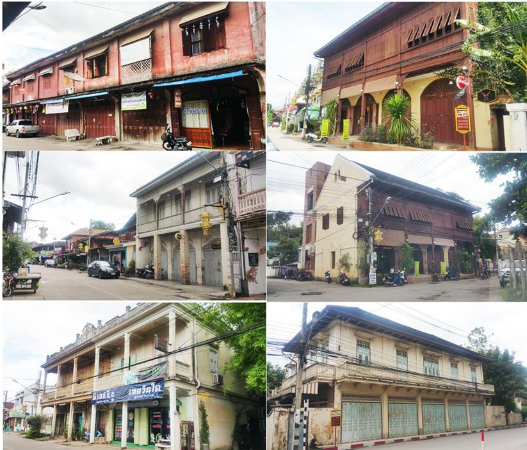
Figure 89 The Old buildings in the Kad Kong Taa area. Source: Em (2016)
