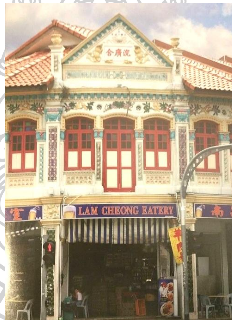
Figure 103 This highly ornamented corner shophouse on Balestier Road encapsulates the quintessence of the Singapore shophouse, with its eclectic mix of Western and Chinese elements.
