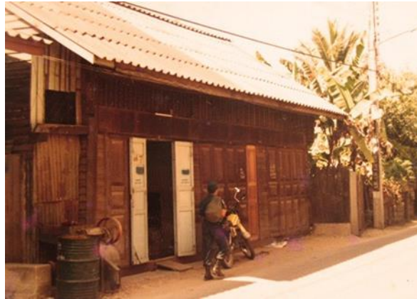
Figure 39 The Riverside 1 restaurant, the old one before being renovated. Source: -
