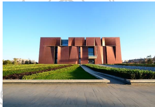
Figure 18 Exterior views of Yunnan Provincial Museum
