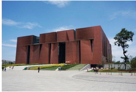
Figure 17 Exterior views of Yunnan Provincial Museum
