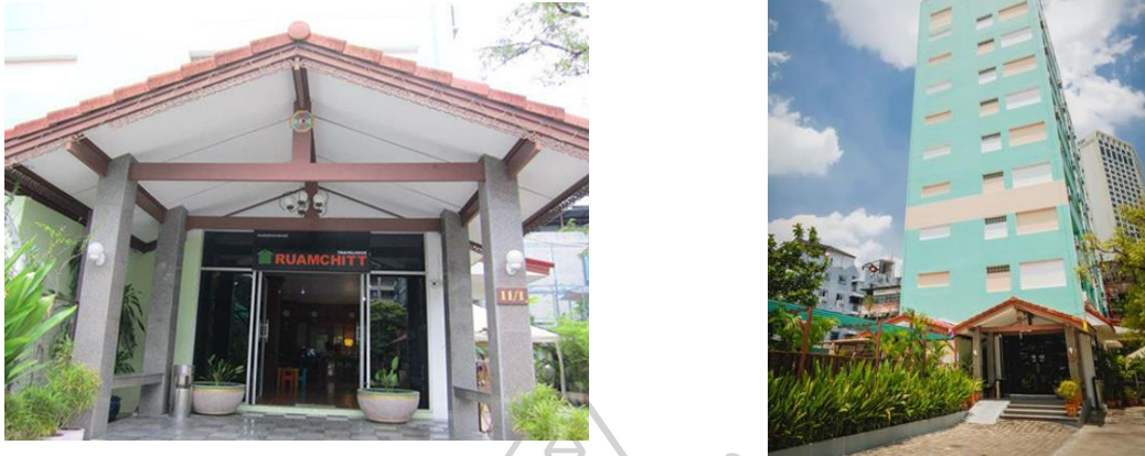
Figure 6 Ruamchitt Travelodge building and entrance
