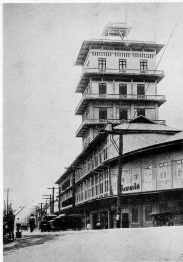
Figure 44 Oldtown Hostel and Nai Lert Building in the past and present Source: www.oldtownhostelbkk.com and Tanat Bha-aryaphatn [2017]
