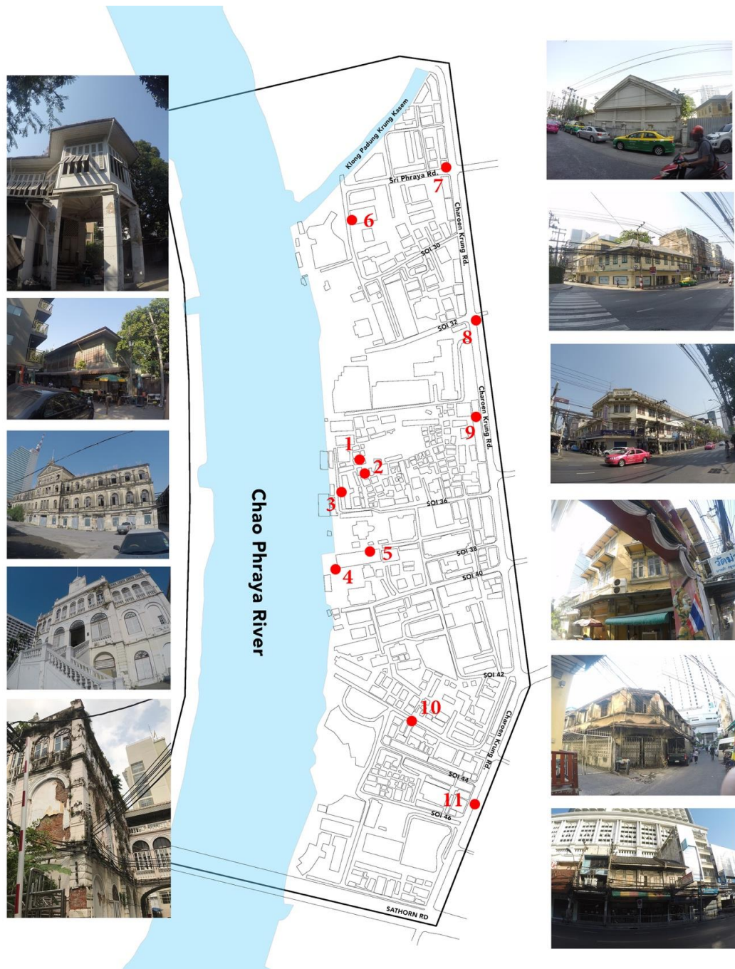
Figure 113 Examples of historic buildings in bad condition Source: Tanat Bha-aryaphatn [2017]
