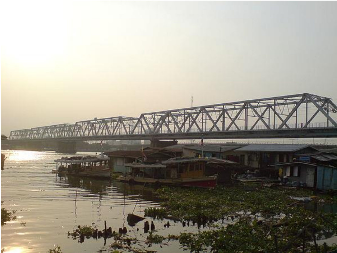
Figure 20 Rama VI Bridge built in 1921
