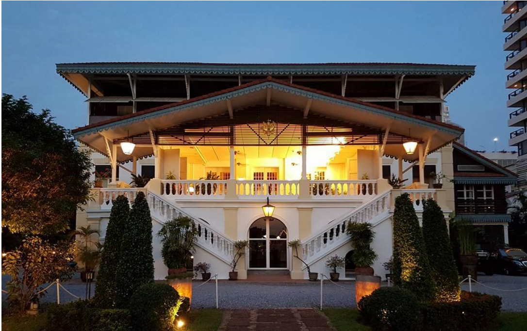
Figure 55 French Embassy original building Source: http://www.bangkokriver.com/th/place/embassy-of-france-bangkok/ [Access 13 January 2017]
