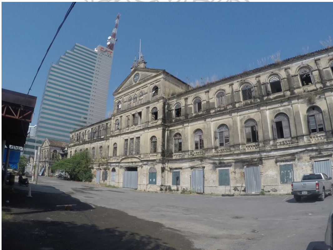
Figure 53 The Old Customs House main three-storey building Source: Tanat Bha-aryaphatn [2017]
