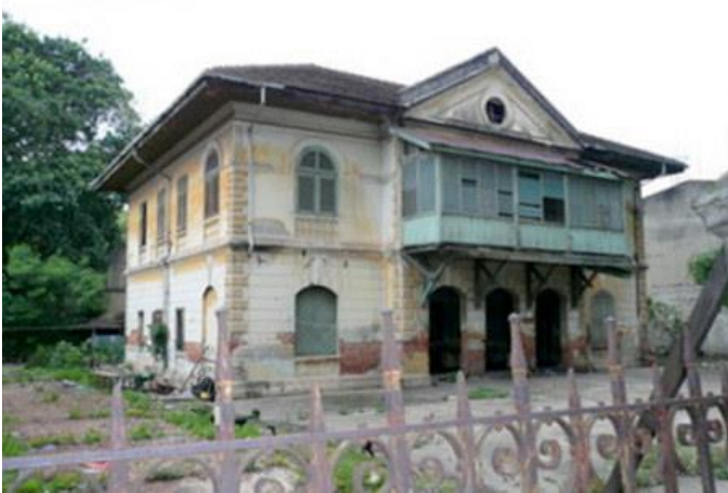
Figure 46 House Number One before renovation
