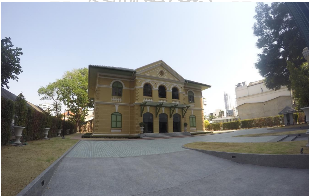
Figure 47 House Number One after renovation completed in 2016
