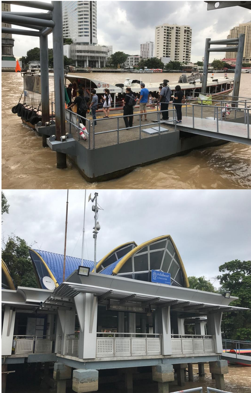
Figure 90 Sri Phraya Pier's existing condition Source: Tanat Bha-aryaphatn [2017]
