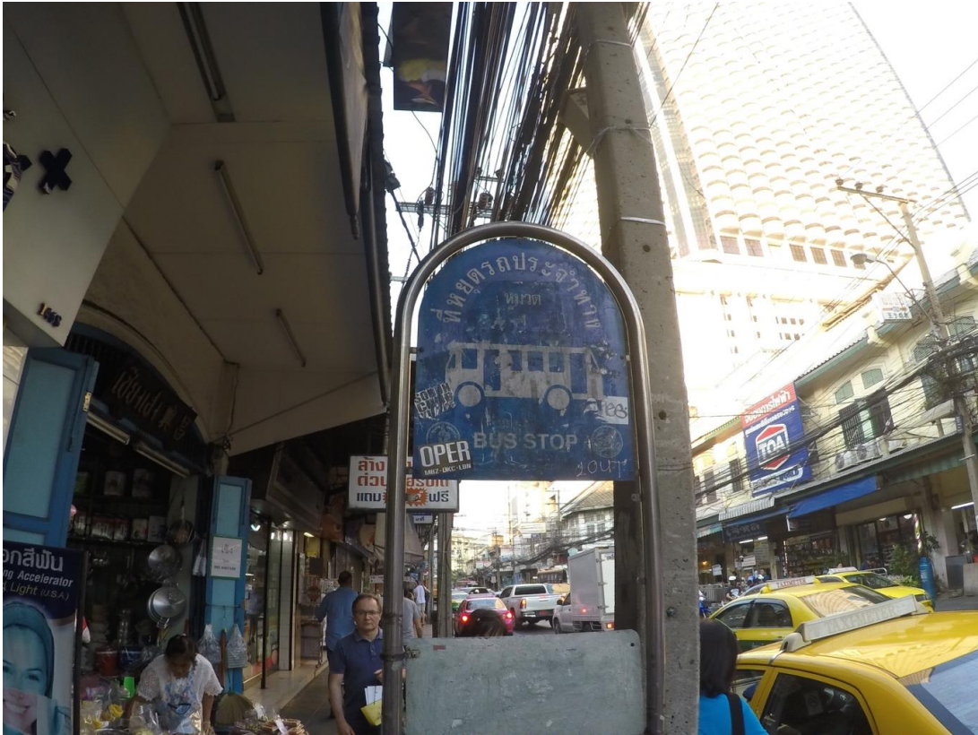
Figure 72 Example of damaged bus stop Source: Tanat Bha-aryaphatn [2017]
