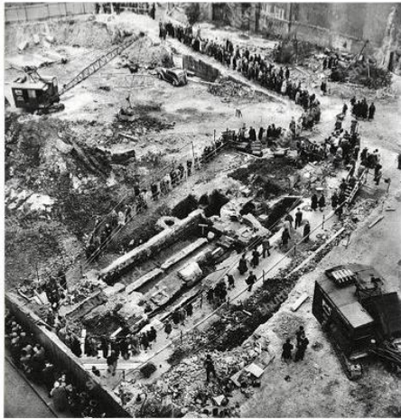
1954 Excavation Temple of Mithras, Walbrook
