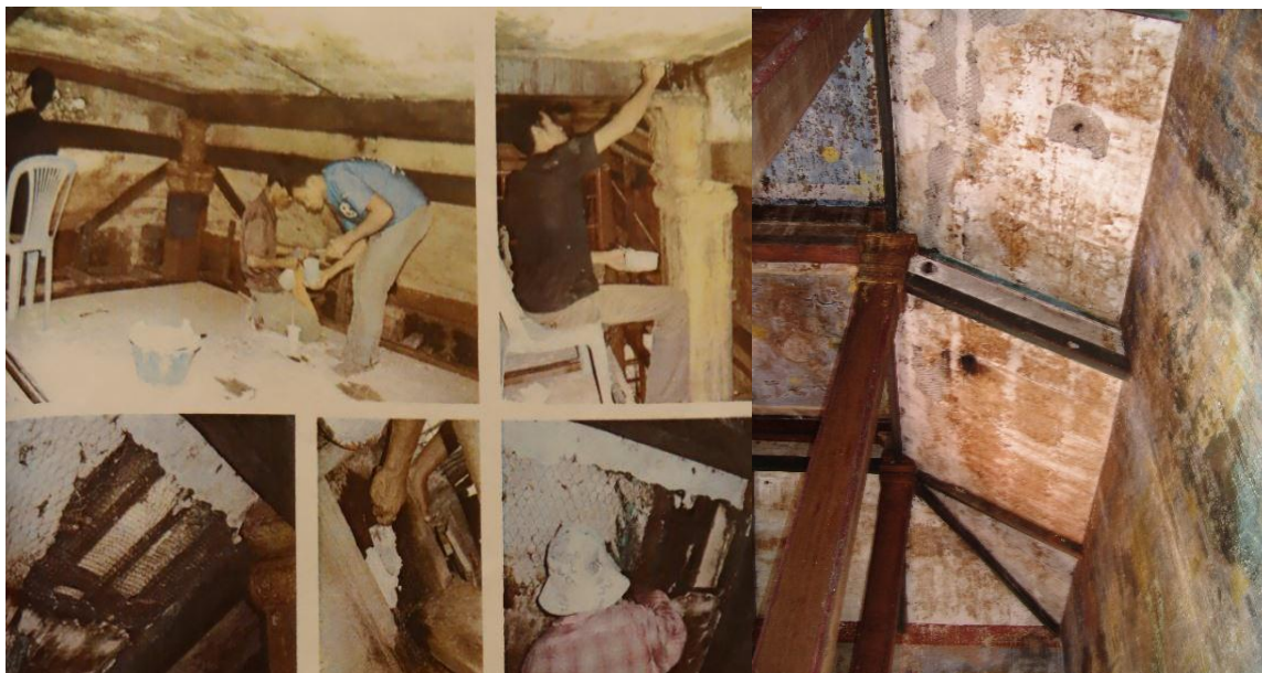
Figure 3 The holes on the roof covering with a net
