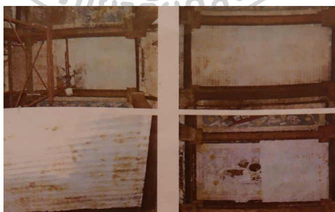
Figure 4 The removed plaster layer with the area of 30 x 60 cm
