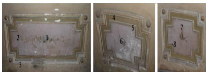
Figure 22 The three mural paintings in El Sakakeny Palace showing sampling points on the damage on the ceiling
