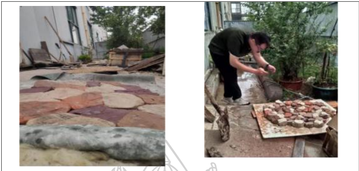
Figure 109 Rainwater scouring (Photographed by Wang Yurong 2020)
