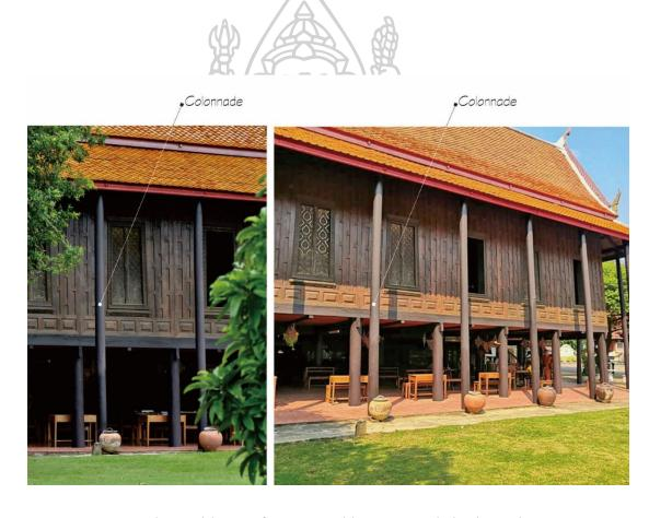
Figure 100 Monk's residence of Wat Kongkharam, Ratchaburi Province a clear example of colonnade archetype created by detaching the column grid out of the wall
