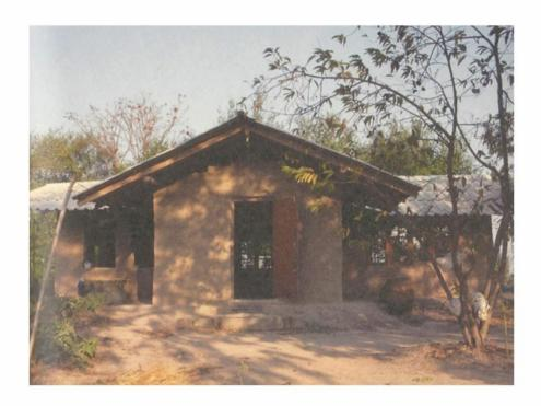
Figure 82 Jon Jandai's own adobe house, costing 7000 baht, under construction Source: Jon Jandai, Yu Kab Din Sibhok Pi Karn Pan Din Pen Baan [16 Years with Clay: Crafting Clay into Home] [in Thai] (Bangkok: Phabphim, 2012), 35.
