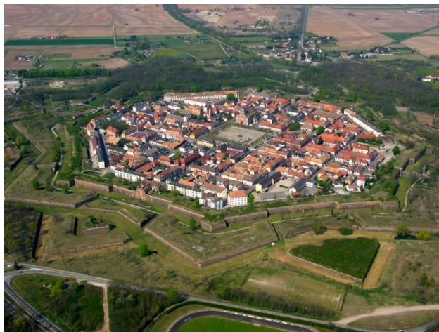
Neuf-Brisach the final fortress designed by Vauban; note how the houses support and reinforce the outer defensive walls 176
