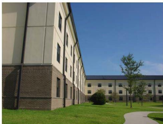
Kessler Air Force Base – Pipeline Dormitory
