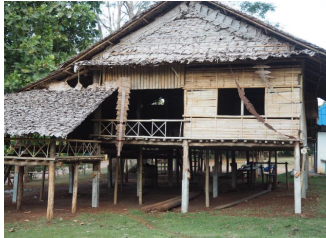
Figure 99: A Karen House in Lin Thin, Thong Pha Phum. House owner shows the pounding tool under the house Source: Author (2019)
