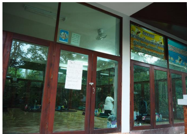
Figure 122: Traditional Thai Massage Building at Hin Dad Hot Spring Source: Author (2018)
