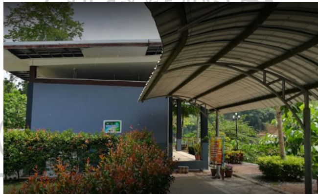
Figure 60: Entrance of building for private spa treatment rooms Source: Phanisa Hualkhogsong (April, 2021)
