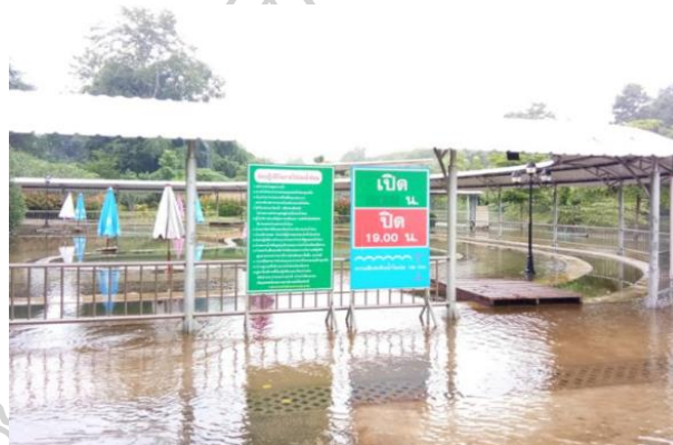
Figure 26: Flooding in Lin Thin in Low Season (August, 2018) Source: https://www.matichon.co.th/news-monitor/news_1077003
