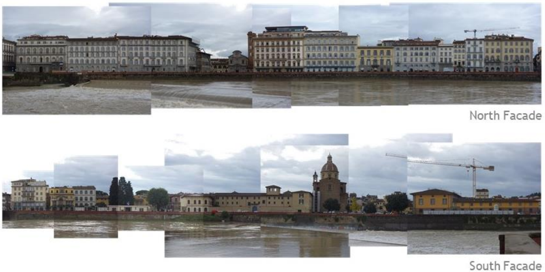
Figure 58. Facade of Arno River
