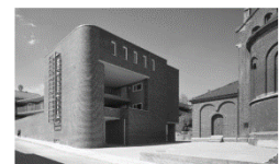
Community centre and senior housing in Stuttgart
