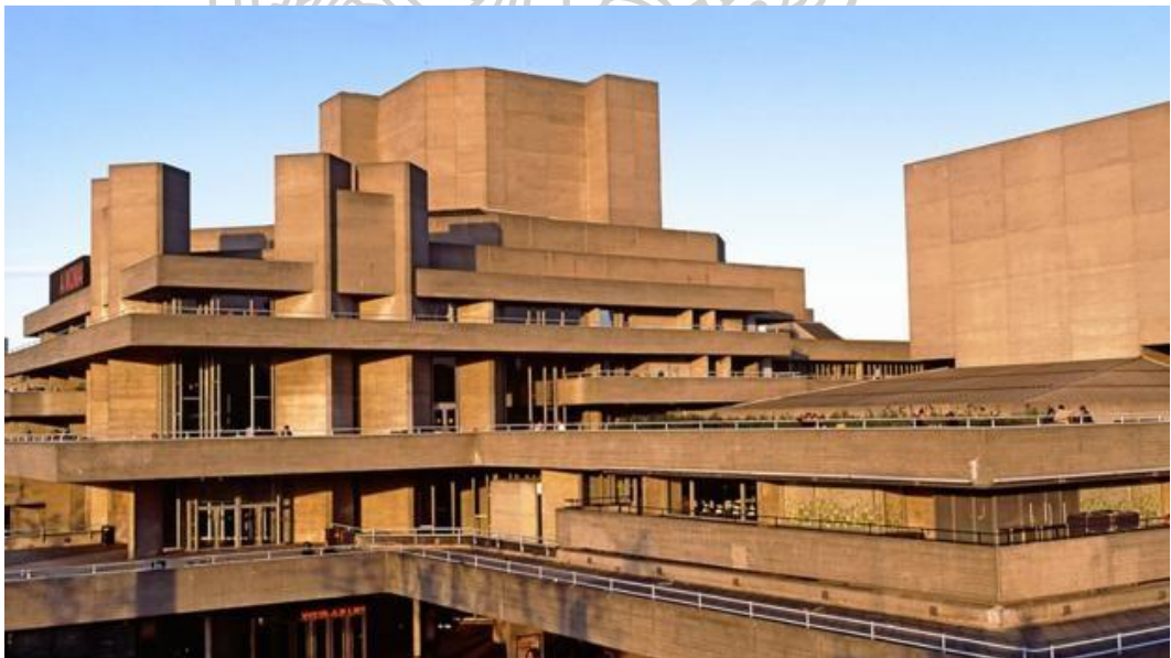
Figure 42 Southbank Centre (Crompton, 1967-1968)
