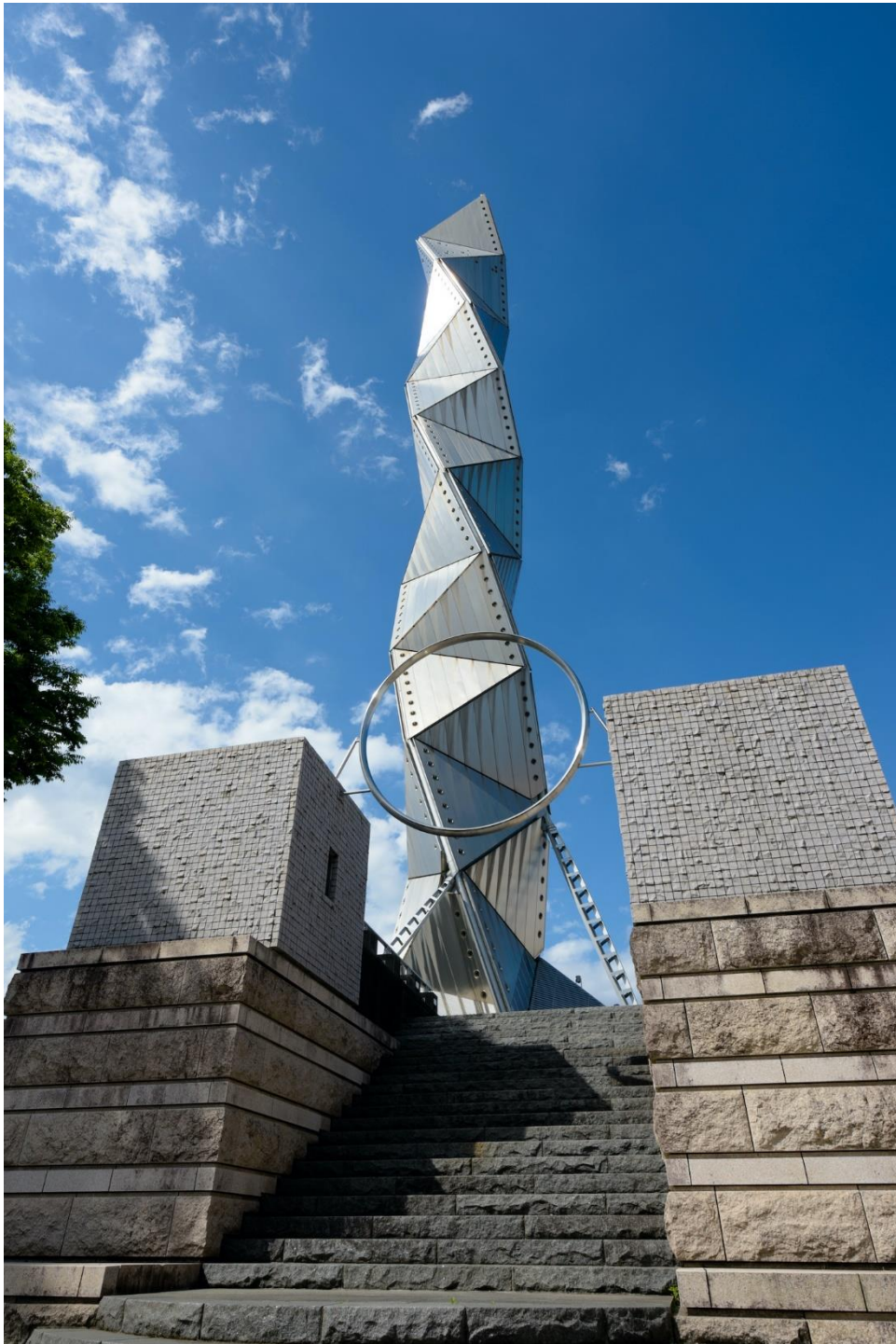
Figure 40 Art Tower Mito, Japan (Isozaki and Associates, 1990)
