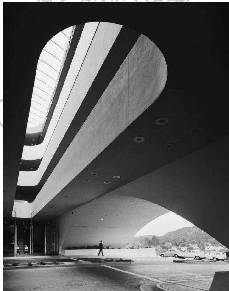
Figure 23 The Marin County Civic Center (1967) in San Rafael by Frank Lloyd Wright,
