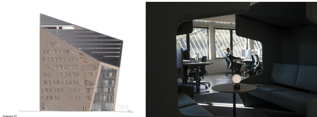
Figure 118 Powerhouse Telemark (Snohetta, 2020) 8
