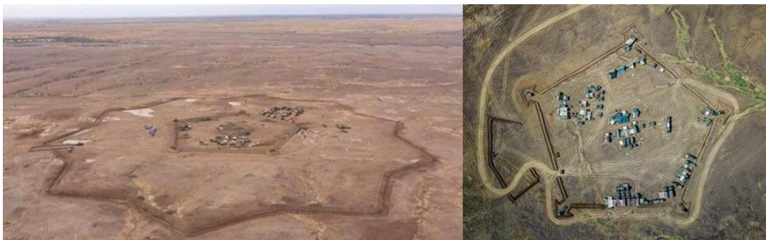
Figure 138. A French military in 2012 base in Mali at Labbezanga (left picture) and Meneka (right picture) which still use Vauban classic fortification layout plan style (Source: https://interestingengineering.com/french-army-revives-medieval-star-fort-patterns-in-north-africa )
