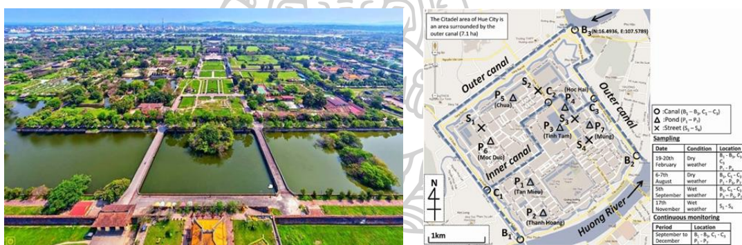
Figure 136. The system of artificial waterways and canals in Vietnamese fortifications ensures the supply of water for the entire city (Source: https://en.wikipedia.org/wiki/Citadel_of_Hue )
