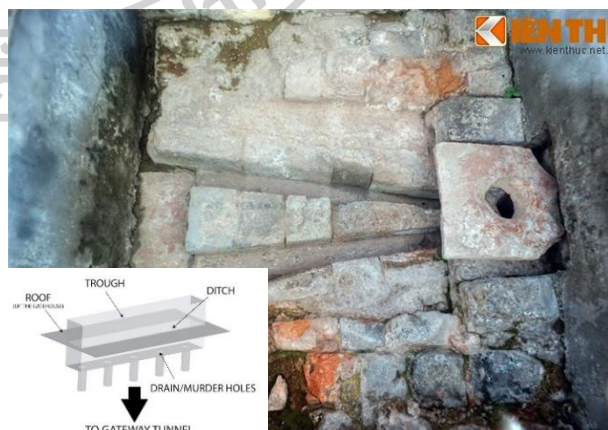
The murder hole of the Thang Long citadel and its supporting slots (Source: kienthuc.net)
