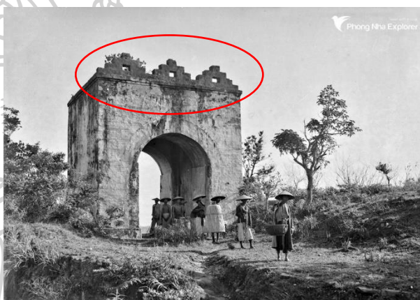
Merlon on Hoành Sơn citadel (built in 1833) (Source: PhongNhaExplorer)
