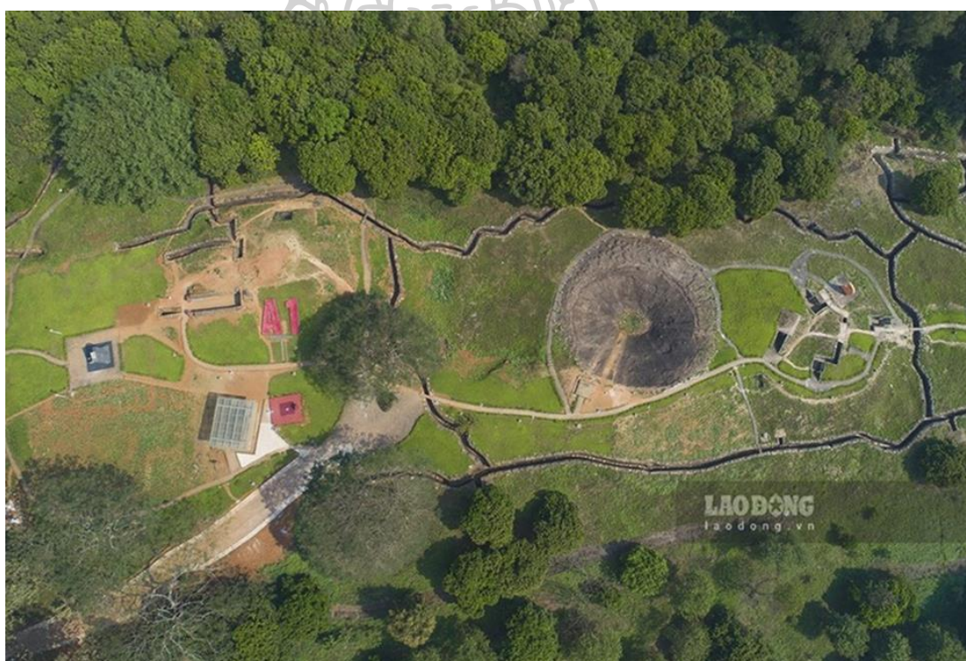
Figure 109. Tunnels and trenches of Dien Bien Phu battlefield between Viet Minh and the French army (Source: laodong.vn )
