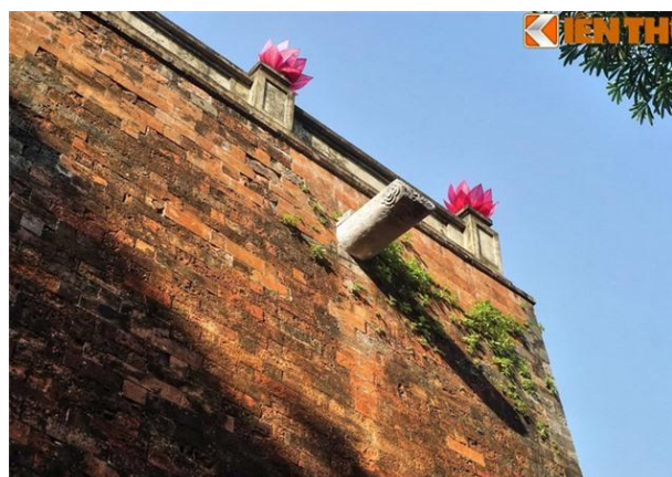
The drain trough of Thang Long citadel (Source: kienthuc.net )
