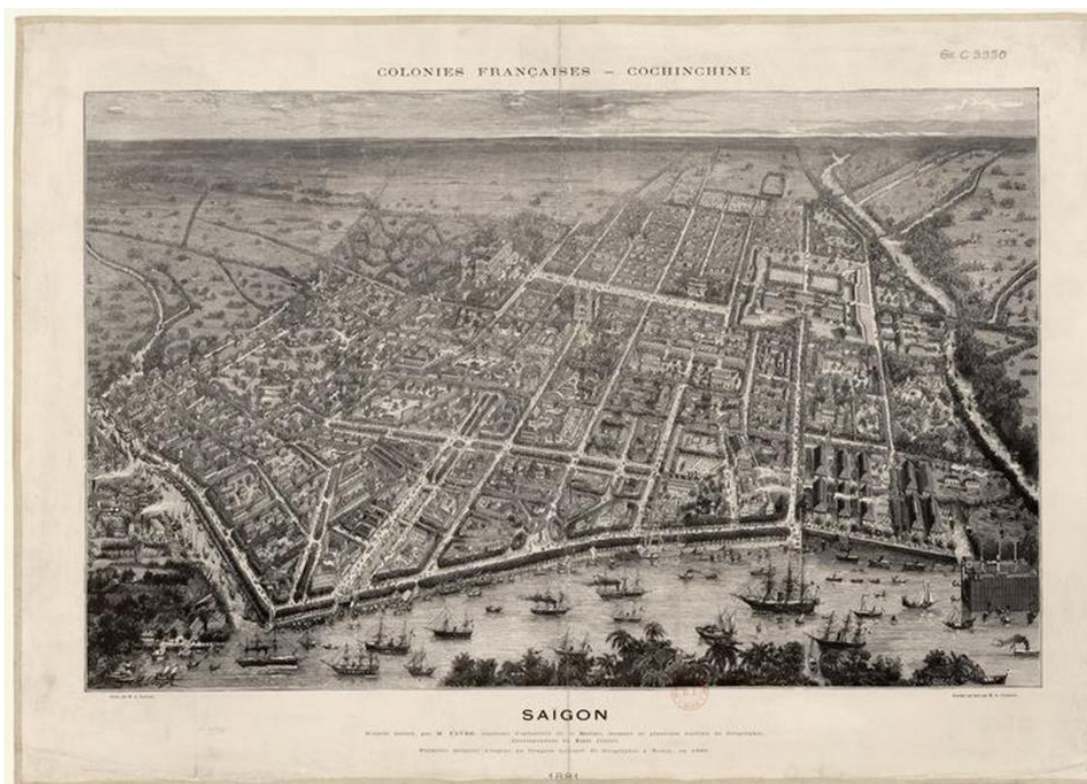
Figure 121. Citadel of Saigon - the first and also the typical example of the Vauban citadel in Vietnam. (Source: https://alchetron.com/cdn/citadel-of-saigon-85aa46a3-d3a2-40ae-a99a-3abdce0aef8-resize-750.jpg )
