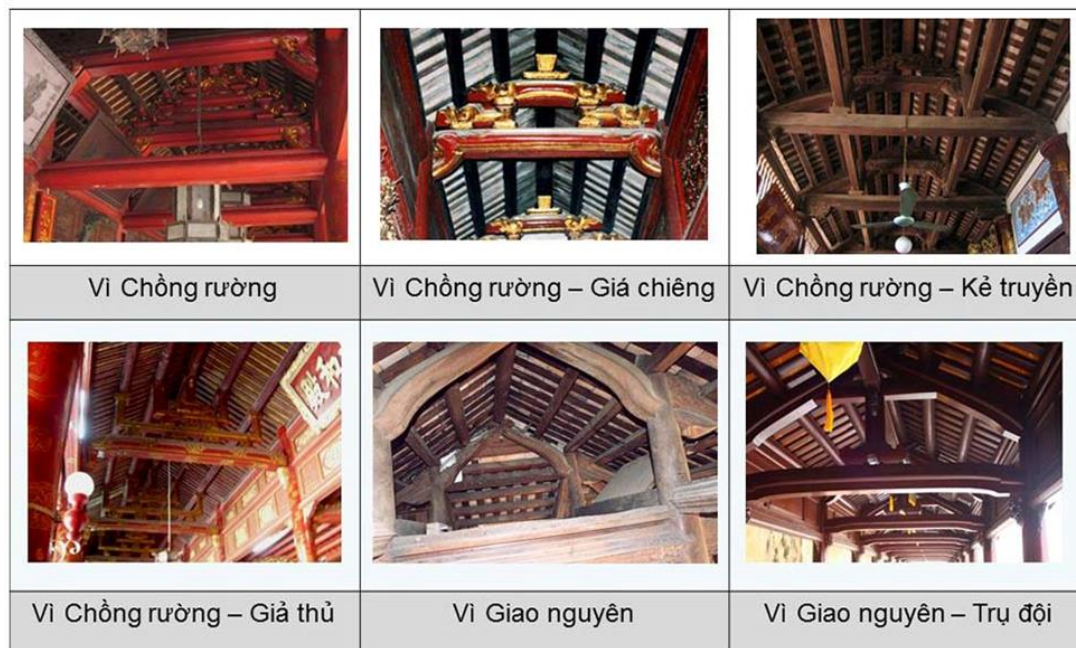
Figure 140. Vietnamese ancient wooden construction techniques are still widely applied to this day
