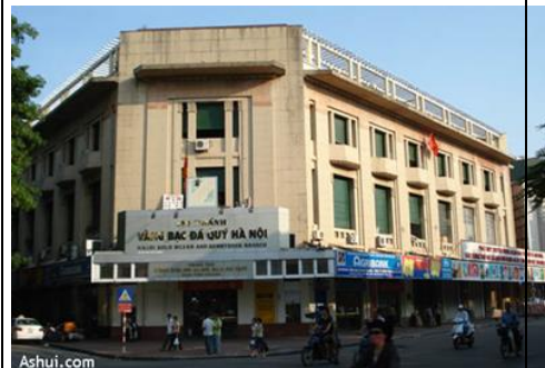
Real estate credit fund headquarters (Source: ashui.com/mag/images/stories/200906/hanoi_artdeco4.jpg )
