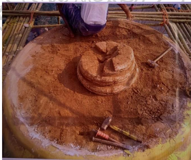
Figure 88: Original Inner Stupa of Moatsotaung Stupa (Under Construction)
