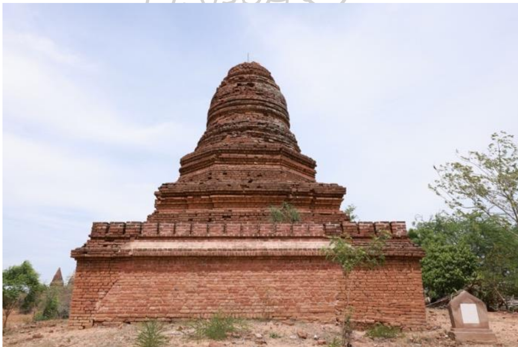
Figure 120: Monument No.329 (Wut-tha-na-daw Group) at the Wetkyi-in Area Note. Inner stupa cannot be seen from the outside after repair by DOA.
