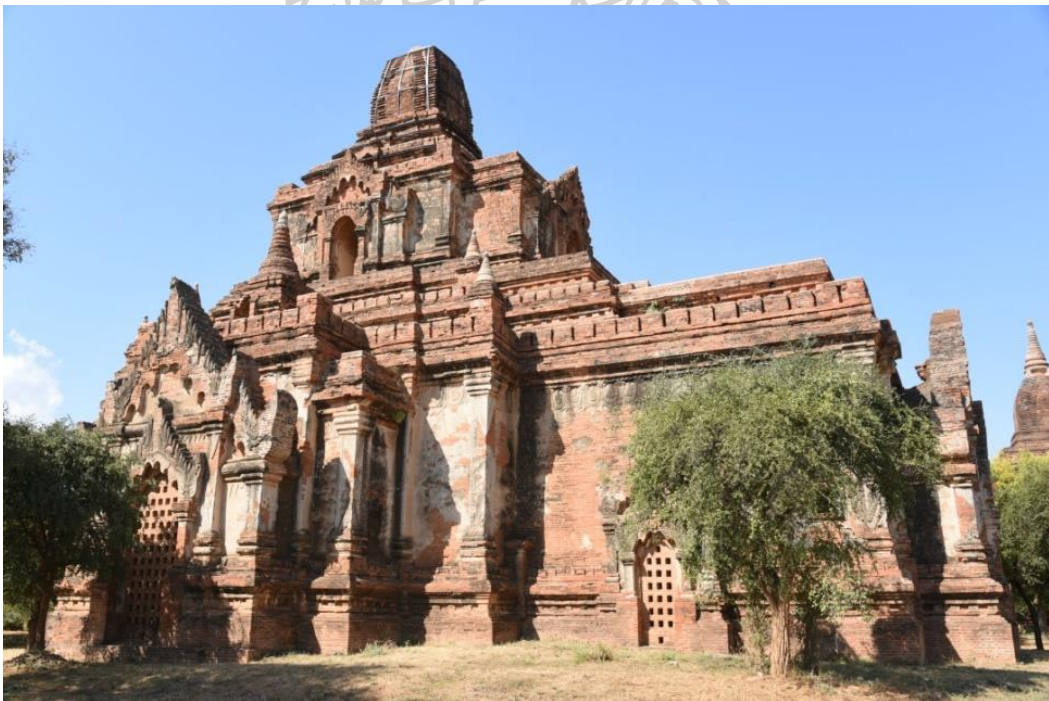
Figure 14: Nwapyagu Temple (No.1498), Two-storeyed Temple, 13 th century CE Note. It is located to the south of Minyeingon Temple in old Bagan area.
