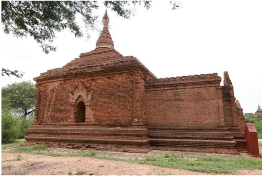
Figure 222: The elevation of the outer temple can be seen here. Note. The inner image house was subsequently enlarged by a larger temple.
