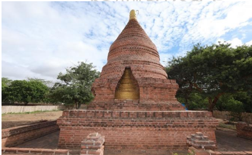
Figure 271: Monument No.1037 at the Thiripyitsaya Area Note. Inner stupa can be visible from the south side.
