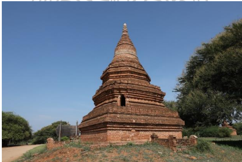
Figure 262: Monument No.1547 at the Myinkaba Area Note. Inner stupa can be seen through a treasure hole at the southeastern corner of outer stupa.
