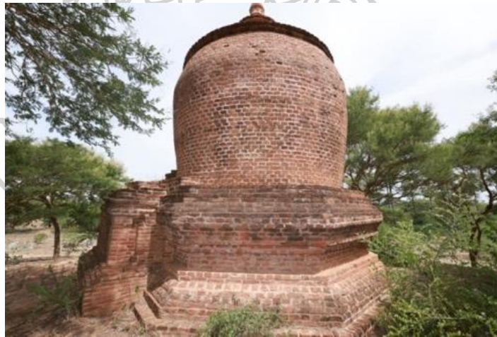
Figure 114: Monument No.280 Viewed from East at the Wetkyi-in Area Note. Inner stupa surmounted with a bulbous-shaped dome can be seen here.
