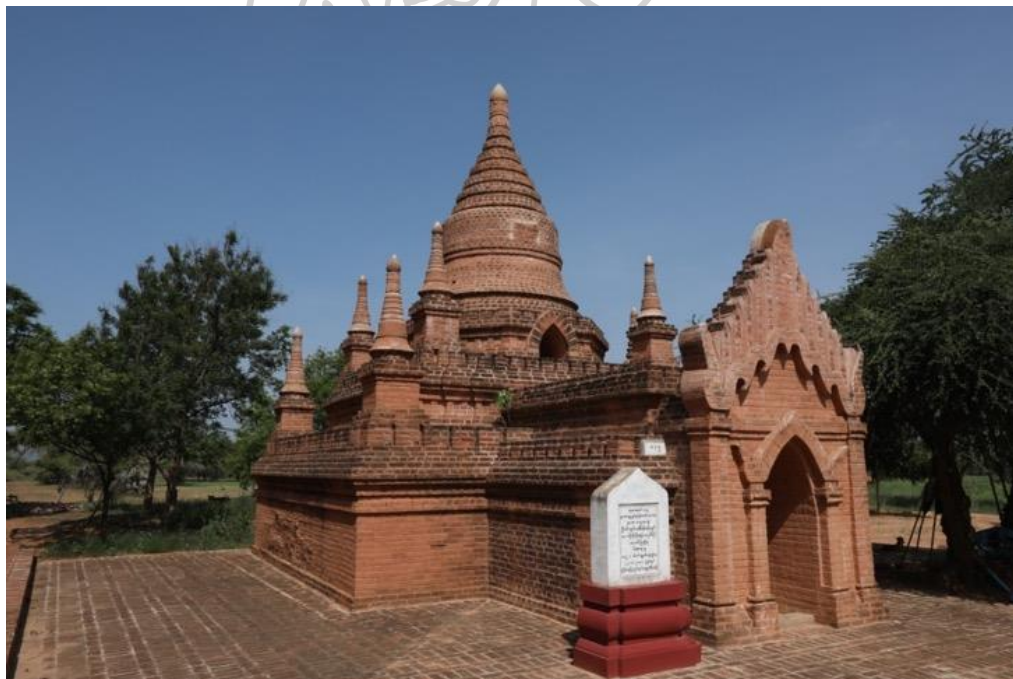
Figure 287: Monument No.819 at the Minnanthu and Phwasaw Areas Note. The inner stupa can be seen from the outside on upper part.
