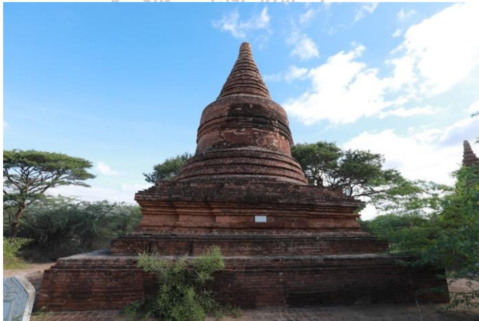
Figure 273: Monument No.1059 at the Thiripyitsaya Area Note. Inner stupa cannot be seen from the outside after repaired by the DOA.
