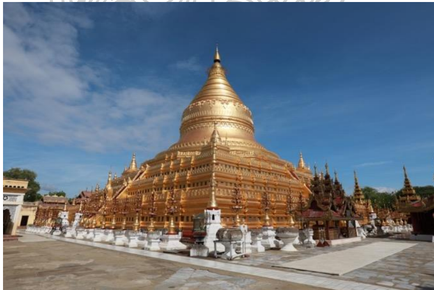
Figure 102: Shwezigon Stupa Viewed from Southeast Direction Note. Three receding terraces with four stairways can be seen in this stupa.
