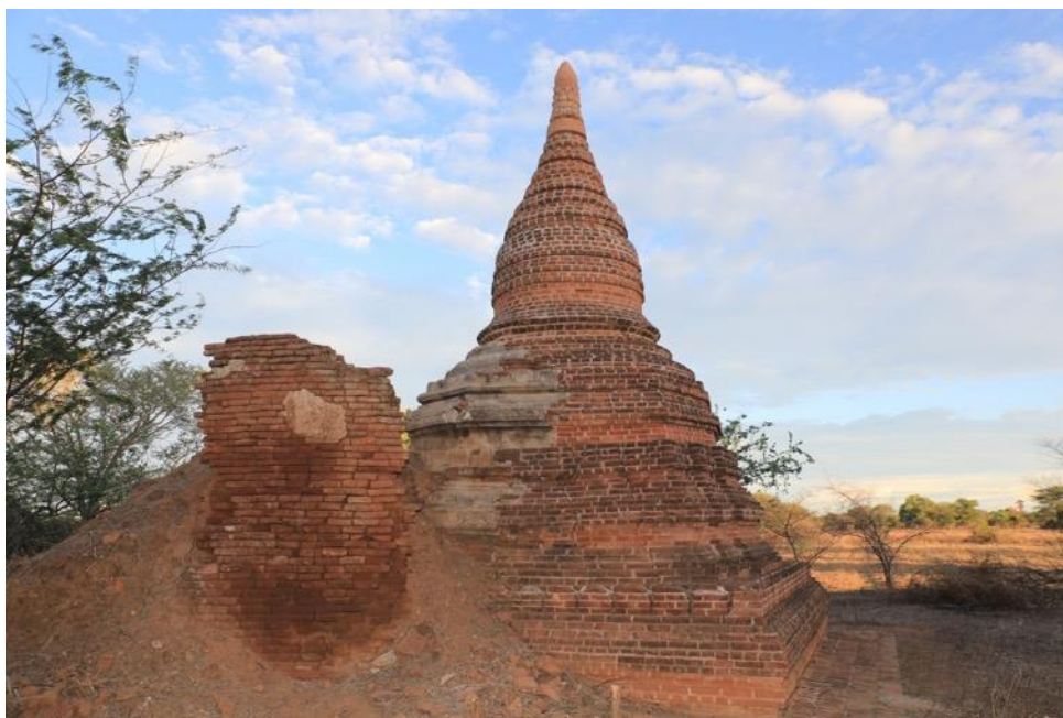
Figure 133: Monument No.445 at the Wetkyi-in Area Note. Outer stupa was not concentrically built around the encased stupa.
