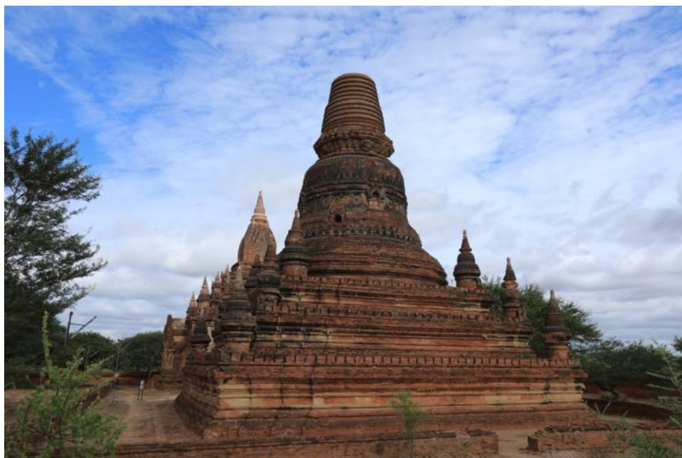
Figure 277: Monument No.1086 (Seinnyet Nyima Stupa) at the Thiripyitsaya Area Note. Top finial of inner stupa can be seen from the southeast side on bell-shaped dome.
