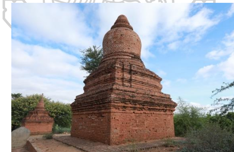
Figure 269: Monument No.1003 at the Thiripyitsaya Area Note. Inner stupa cannot be seen from the outside after being repaired by the DOA.
