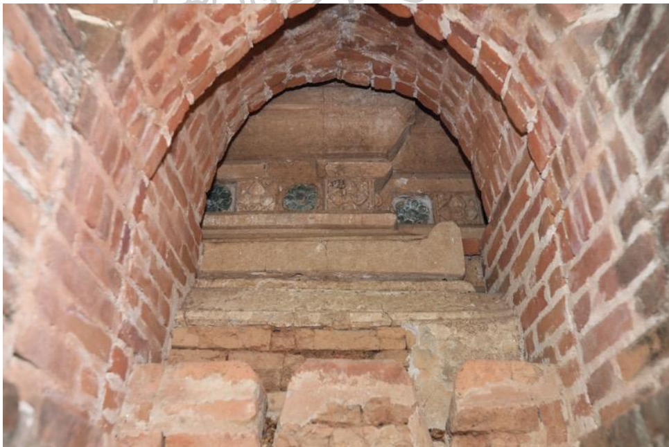
Figure 258: There is a niche exposed to see and worship the inner stupa here. Note. Original glazed and stucco decorations on the encased stupa can be seen here.
