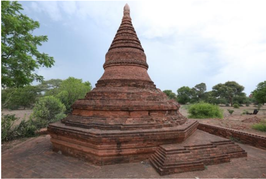
Figure 153: Monument No.1697 at the Taungbi Area Note. A part of outer stupa still remains at the southeast corner of inner stupa.
