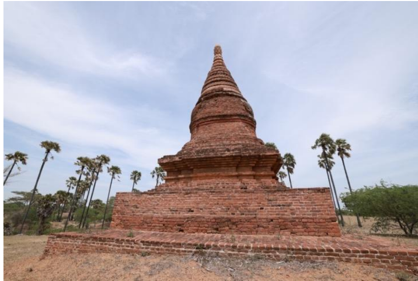
Figure 112: Monument No.272 at the Wetkyi-in Area Note. Inner stupa is not visible from the outside after repair by DOA.
