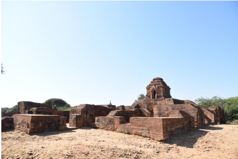
Figure 26: Somingyi Monastery (No.1147), Monastery with multiple cells around the main hall, 12 th century CE Note. It is located to the south of Somingyi Stupa, south of Myinkaba Village.
