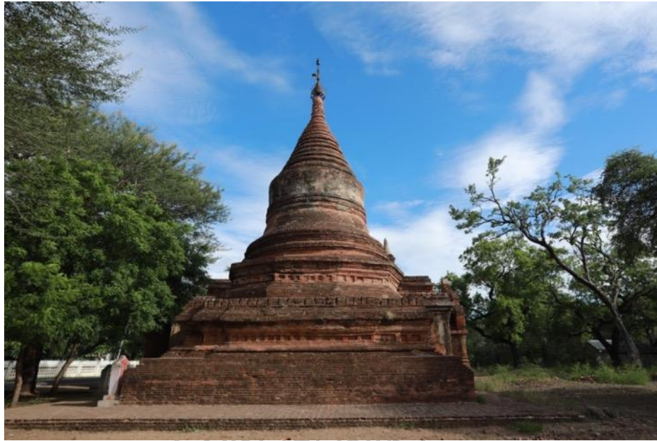
Figure 214: Monument No.1666 at the Old Bagan Area Note. Inner stupa cannot be seen from the outside after repair by the DOA.
