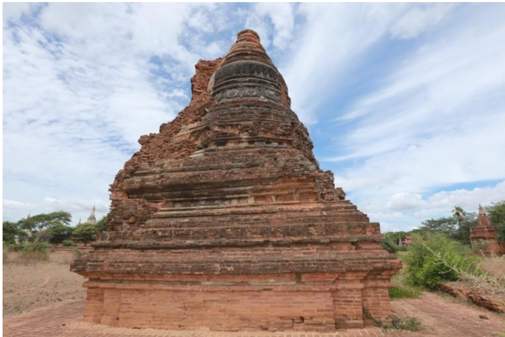
Figure 175: Monument No.1905 at the Taungbi Area Note. There is no space between the inner and outer stupas.
