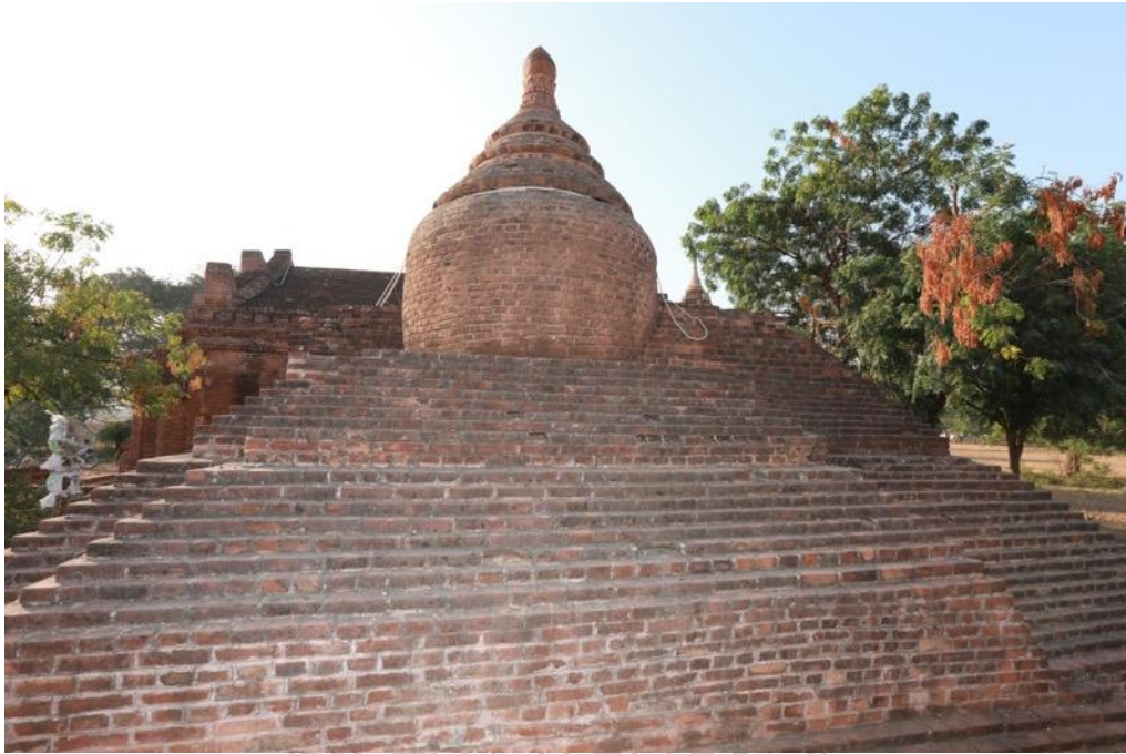
Figure 255 Monument No.1456 at the Myinkaba Area Note. Inner stupa with bulbous-shaped dome can be seen from the outside here.
