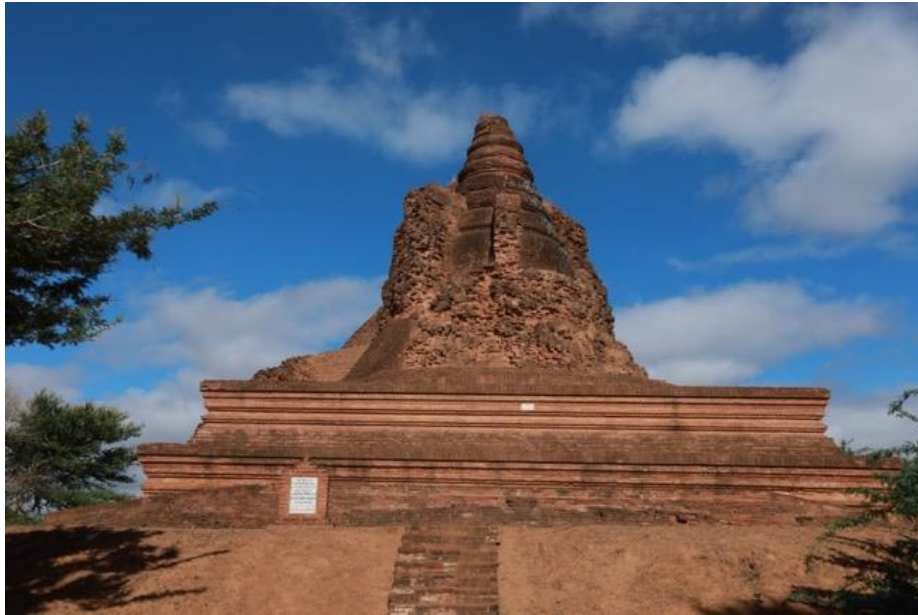
Figure 220: Monument No.1158 (Kyauk Myet Maw Stupa) at the Myinkaba Area Note. The radiating walls around the inner stupa can be seen here.
