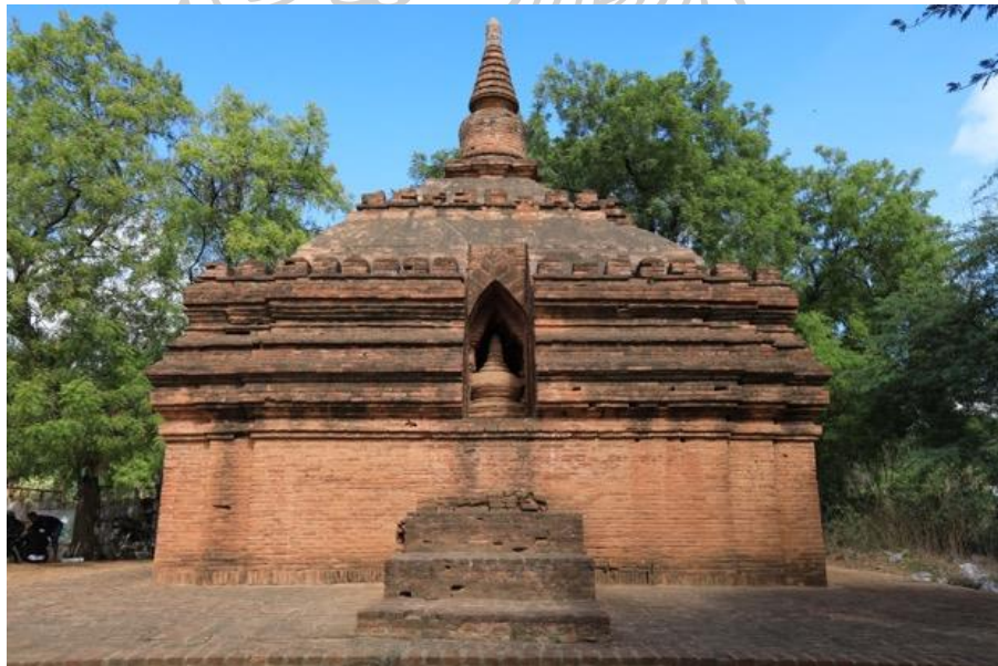
Figure 237: Monument No.1225 at Myinkaba Area Note. Half portion of inner stupa is located in the eastern wall of outer temple.
