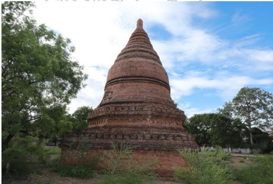
Figure 212: Monument No.1663 at the Old Bagan Area Note. The inner stupa cannot be seen after repair by the DOA.
