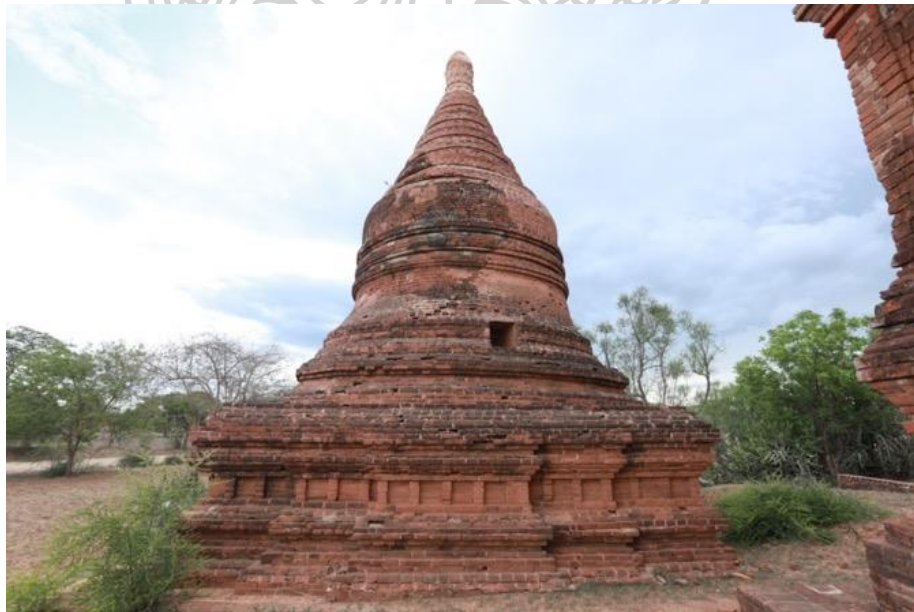
Figure 151: Monument No.1696 at the Taungbi Area
