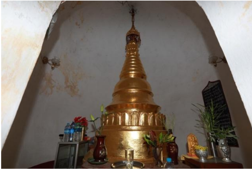
Figure 105: Original Gilded Inner Stupa at the Nyaung U Area Note. The space between inner and outer structures is seen here.
