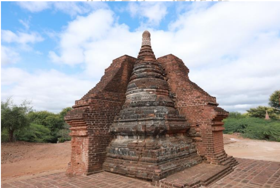
Figure 217: Monument No.1155 at the Myinkaba Area Note. Inner stupa with original stucco decorations can be seen here.
