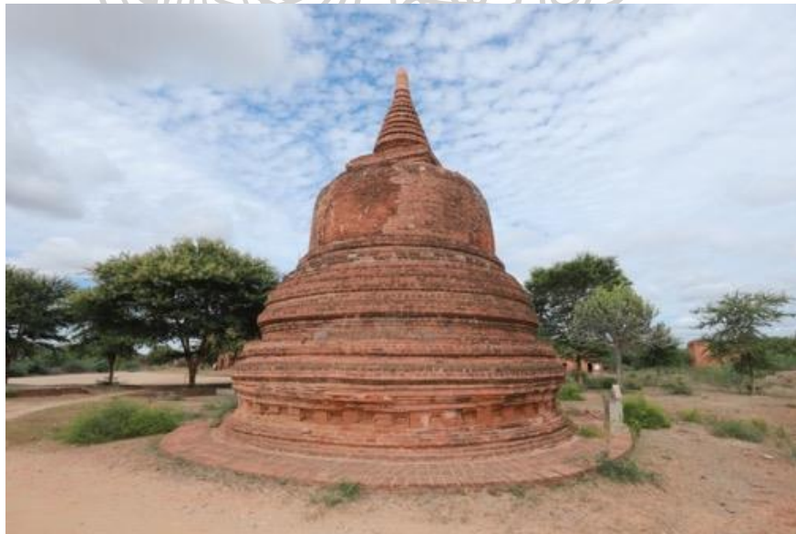
Figure 157: Monument No.1722 (Sinhalese-Typed Stupa) at Taungbi Area Note. Inner stupa cannot be seen from the outside after repaired by the DOA.
