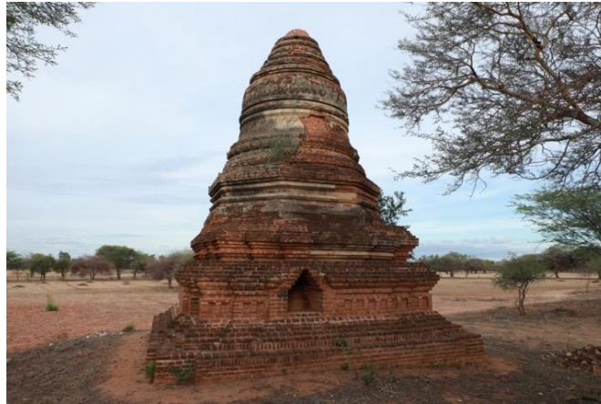
Figure 285: Monument No.805 at Minnanthu and Phwasaw Area Note. Inner stupa can be seen from the outside in this stupa.
