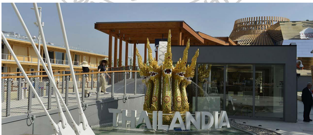
Figure 51: Thai Pavilion at the World Expo Milan, Italy, 2015 (Bureau International de Expositions (BIE), 2015-a)
