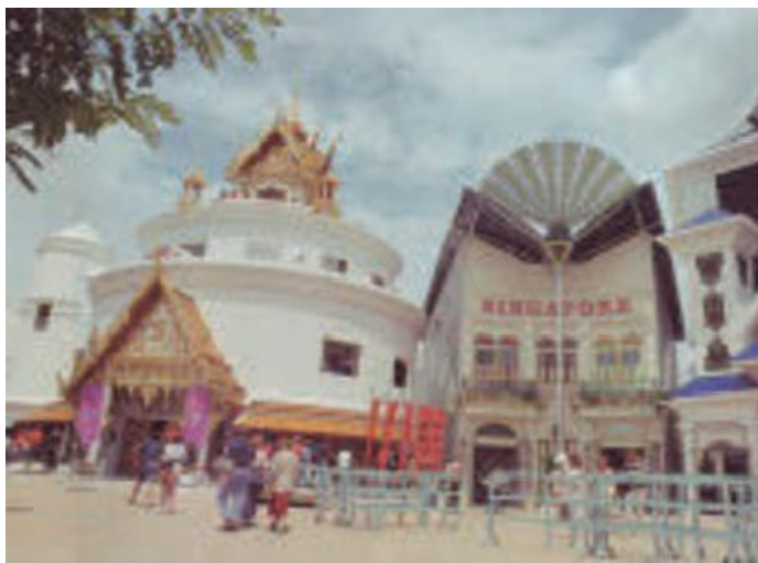
Figure 84: Thai Pavilion, World Expo, Sevilla Spain 1992 (ASA 24, 1992: 34, as cited in Horayangkura, 2010)
