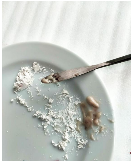
Figure 55, Figure 56: Mixing the filling material and filling the cracks using a spatula.
