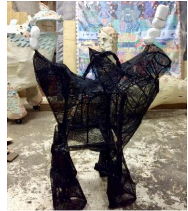
Figure 26. The iron support is covered by hexagonal plastic netting before starting the stucco process. Source: Thaworn Kwamsawat
