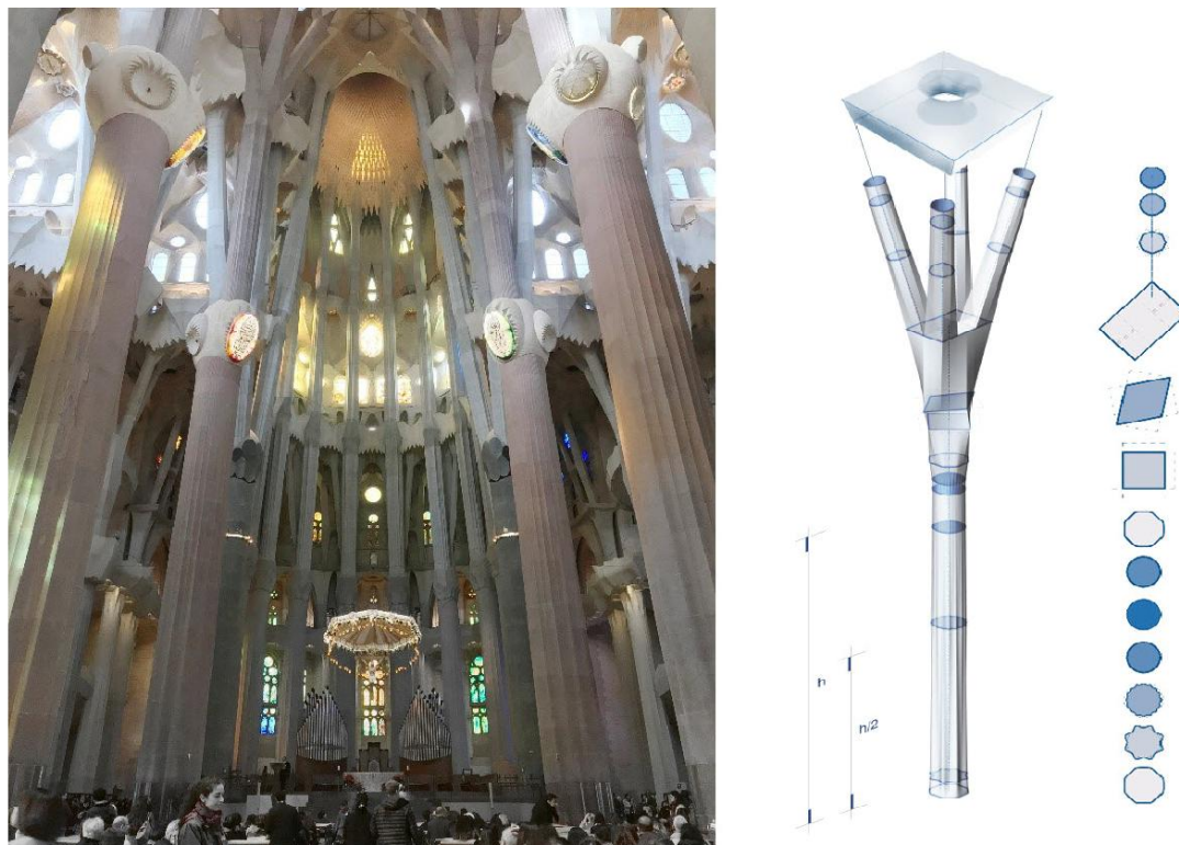
ภาพที่ 35 Geometric Shape, Structure and Material in Antoni Gaudi's Work: The Colònia Güell Crypt and the Templo Expiatorio de la Sagrada Familia (Left) the central atrium of the church; (right) pillar construction scheme.
