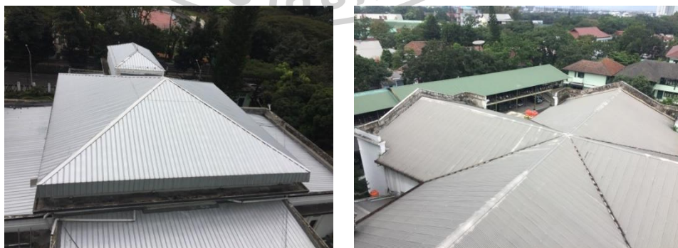
Figure 47 Main building roof (left) and exhibition building roof (right)
