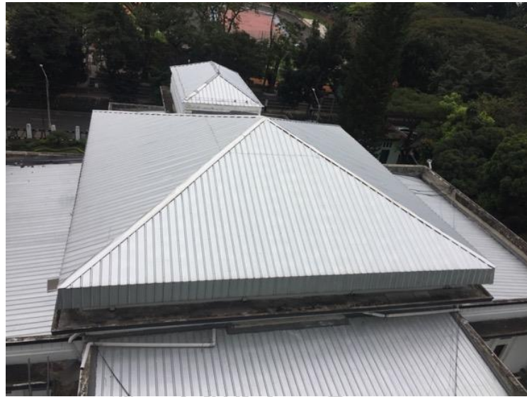
Figure 24 Main Building Roof with New Material and Construction Source: Private, 2022
