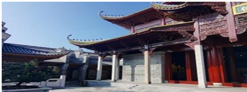
(1) Xu Xun Hall Main Building
