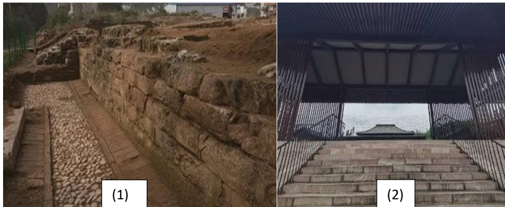
Figure 56 Dragon-Tiger Gate before and after the Protection Project Source: (1) National Cultural Heritage Administration China, n.d.; (2) Author
