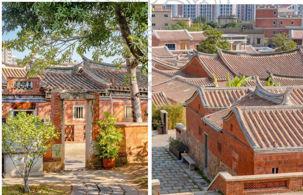
Figure 7: Traditional architecture of southern Fujian
