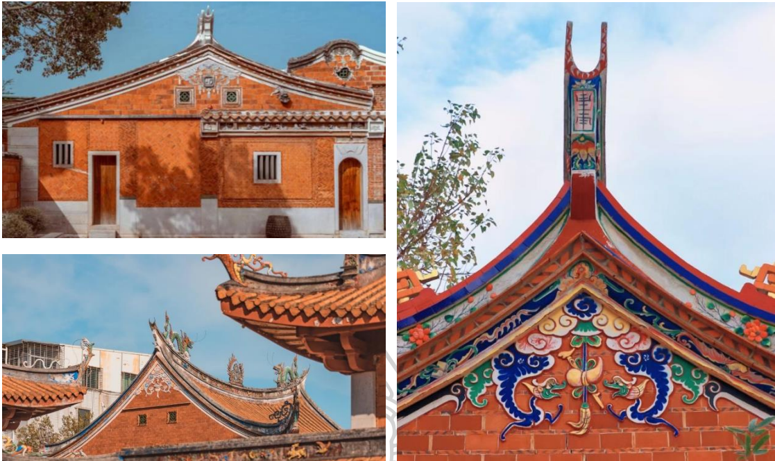
Figure 35: Southern Fujian Roof - swallowtail ridge
