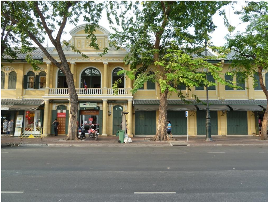
Figure 46 Na Phra Lan shophouses terraces after restoration.
