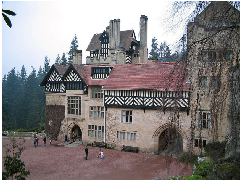
Figure 7 Cragside, Northumberland, 1869. Architect Richard Norman Shaw.
