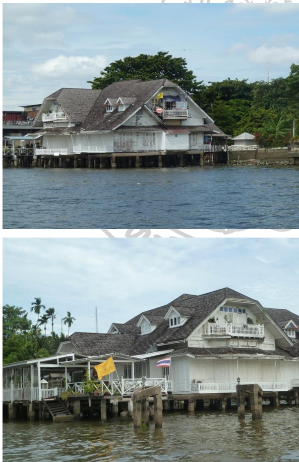
Figure 18 Two examples on the Chao Phraya riverbank: Timber frame construction, roof forms are hybrid hip-and-gable, dormer windows. Roof coverings are kite tiles.
