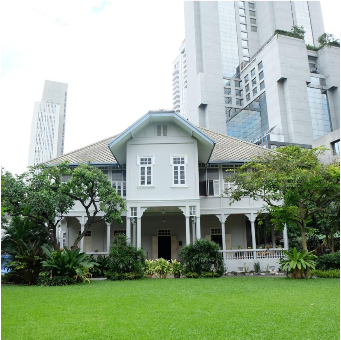
Figure 23 The Rama VI style house at 19 South Sathorn Road. The garden space and its extent is as much part of the Rama VI aura as the house itself.
