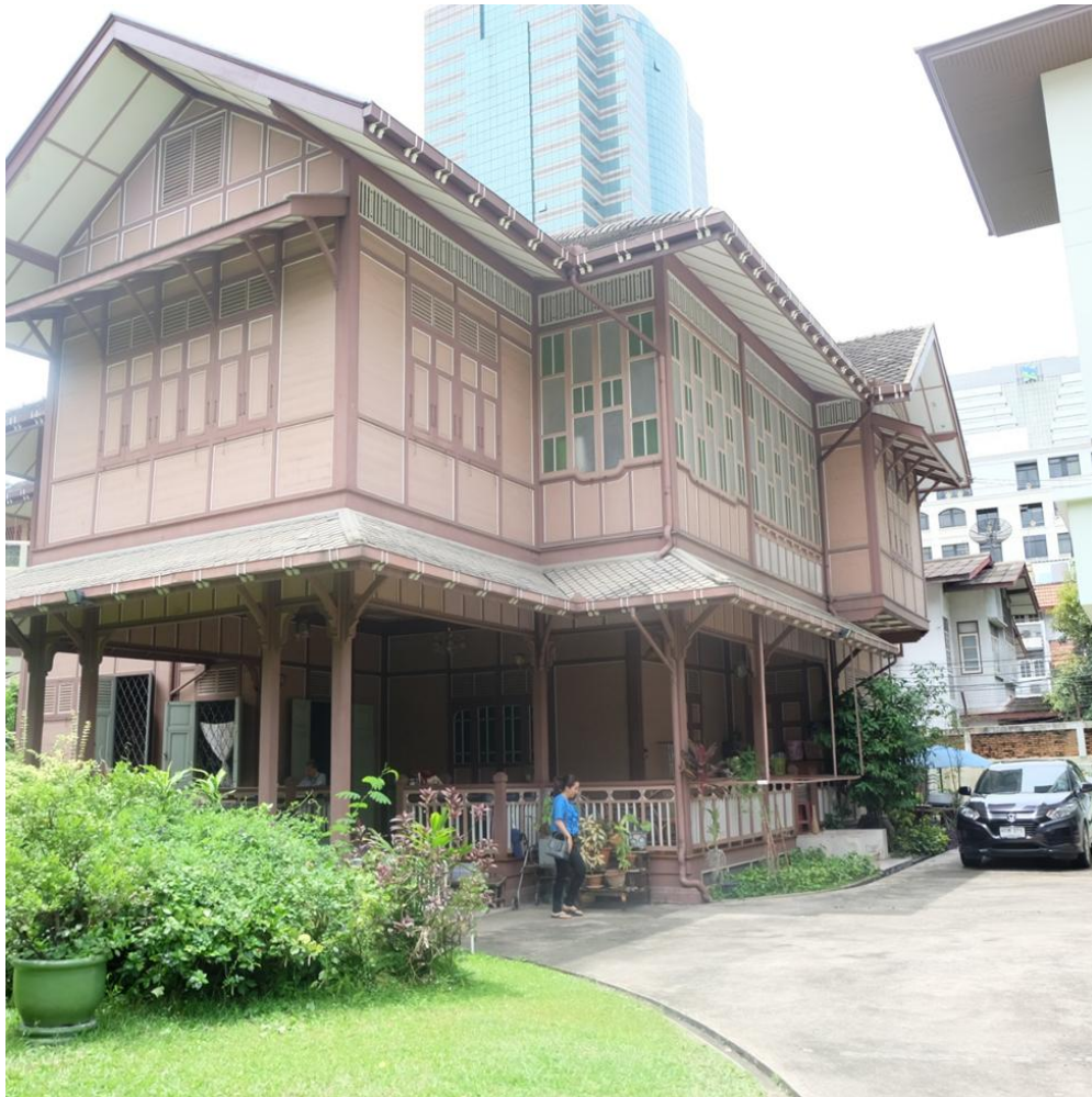
Figure 31 The under-storey as a veranda. Note the complexity of glass panes on the upper store, revealing the affluence of the house's provision.
