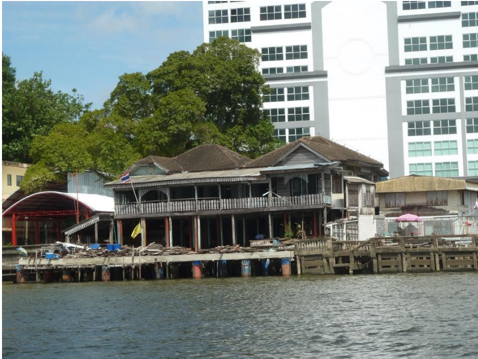
Figure 19 Again timber frame construction. Complex roof forms, both gable and hybrid hip-and-gable, kite tiles. Complex use of decorative timber fretwork. Verandas are typical of the style.
