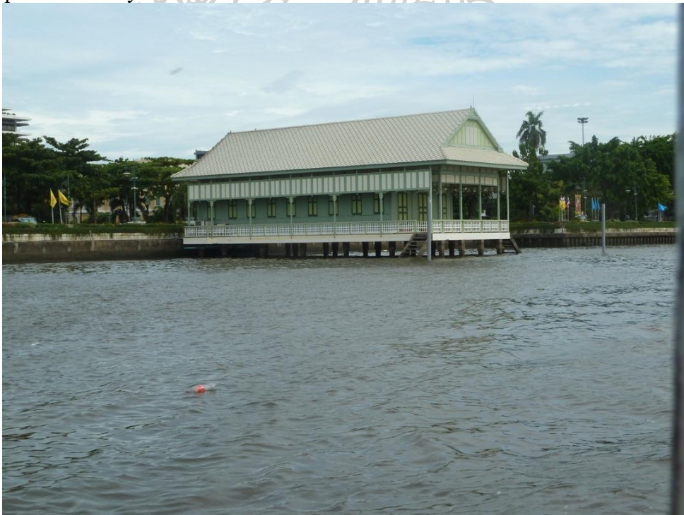
Figure 20 A simpler example: timber frame, hybrid hip-and-gable roof, kite tiles, decorative timber fretwork.
