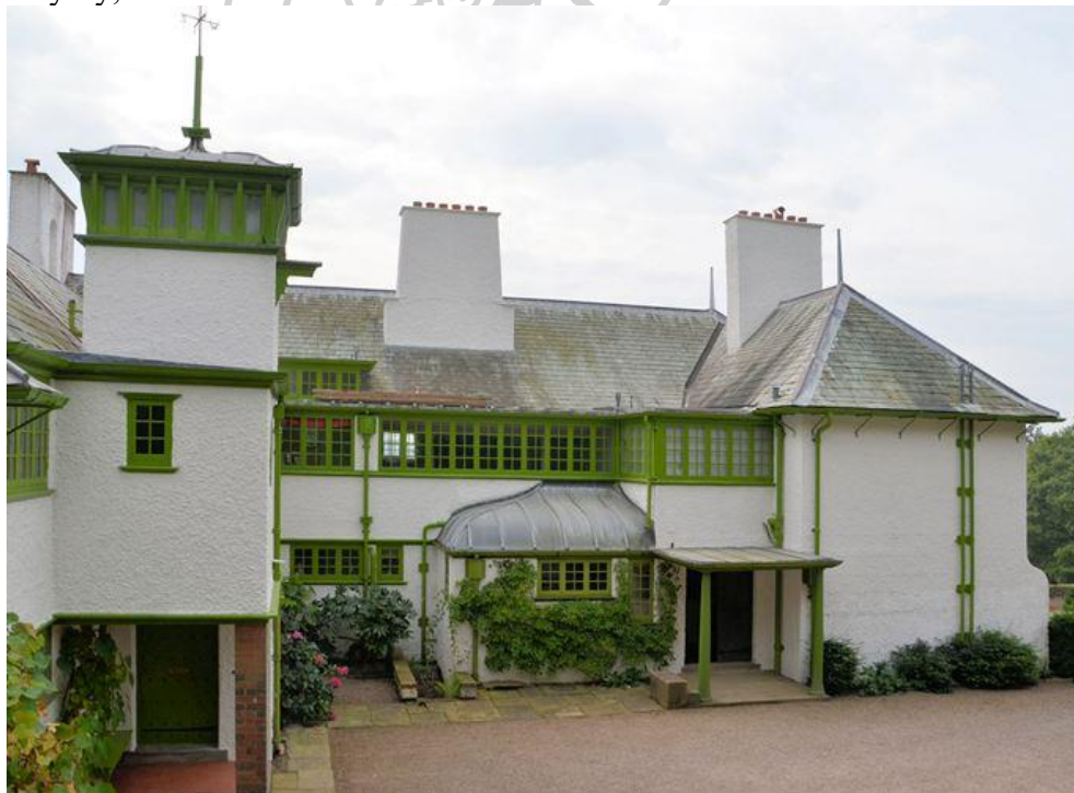
Figure 9 Perrycroft, Colwall, Malvern. Architect C.F.A. Voysey, 1893.
