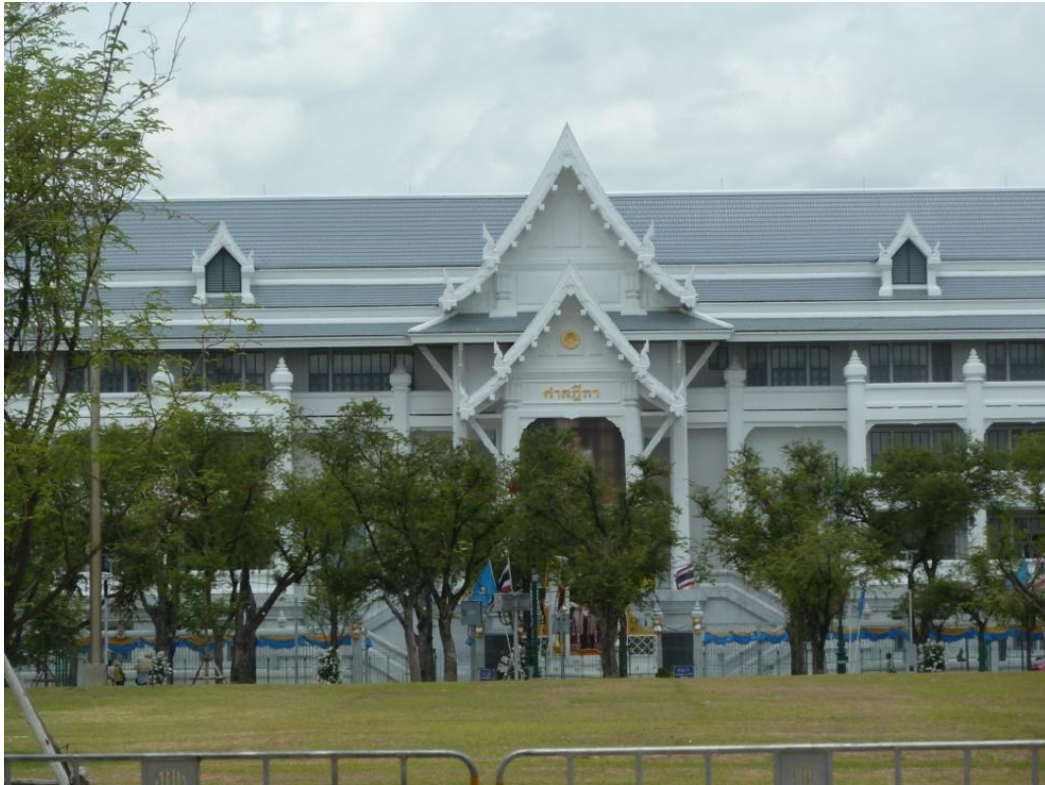
Figure 49 The new Supreme Court building
