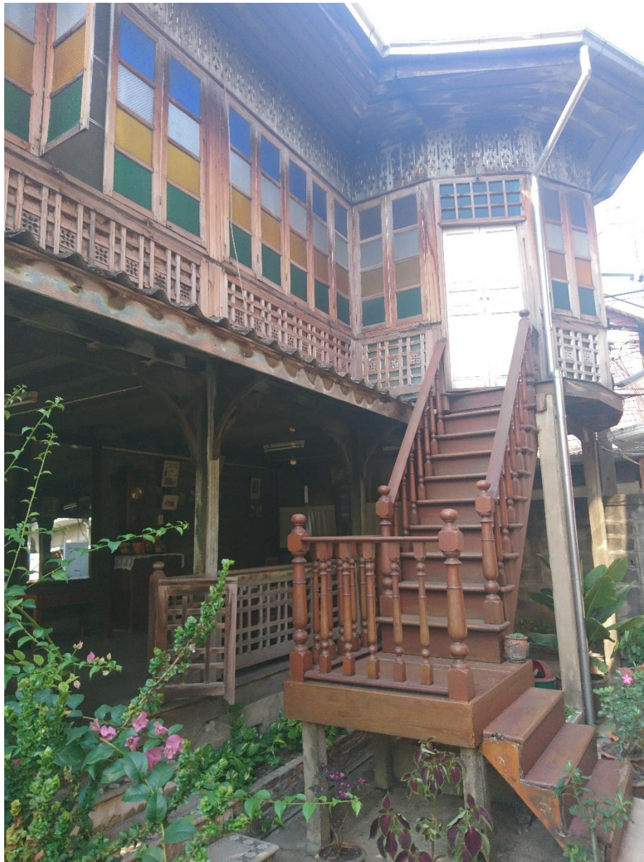
Figure 37 A traditional wooden house from the Rama VI era located in the Ban Krua Nuea community, Bangkok. The structure exemplifies key architectural features of the period, including a raised wooden platform, elaborately carved fretwork panels, and multicolored glass windows arranged in vertical strips. The external staircase and elevated design reflect vernacular adaptations to the tropical climate. This house serves as a living testament to early 20th-century middle-class domestic architecture and the persistence of cultural memory in a rapidly modernizing city.
