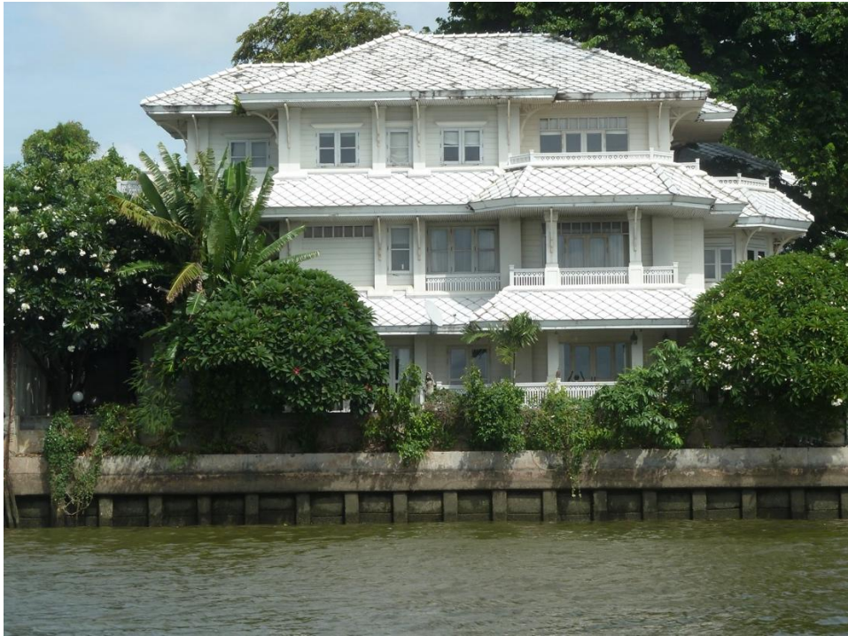
Figure 21 Roofs and cantilevered window hoods are in hip form, again with kite tiles. Note the use of strutted eaves cantilevers on the upper storey.
