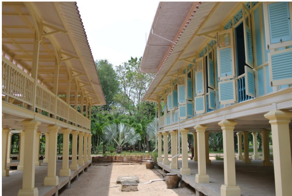
Figure 16 Mrigadayavan, Seaside Palace of King Vajiravudh, Rama VI: the search for a distinctively Thai (and un-Chinese) modernity (source: Sompong Amnuay-ngerntra)
