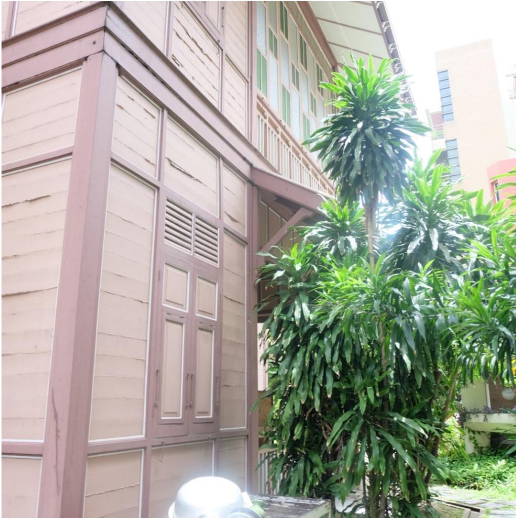
Figure 28 Detail of fine timber work. Note the elaborated window shutters.
