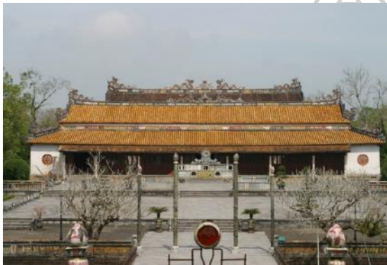
Figure 26: “Thai Hoa Dien” palace in Hue Imperial City, built in 1805 (Source: http://vietnam.lah-waseda.jp/history_4.html )
