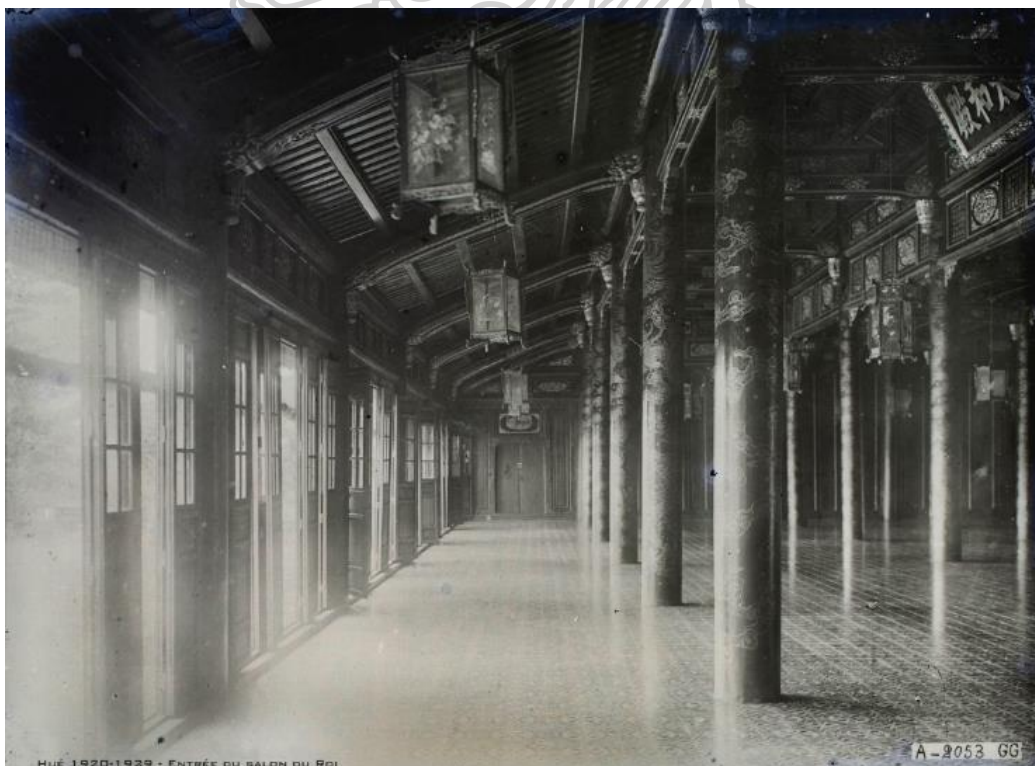
Figure 80a) The interior photos of “Thai Hoa Dien” palace (1920-1929) (Source: https://www.flickr.com/photos/13476480@N07/46849663681/ ) Date of access: September 2021
