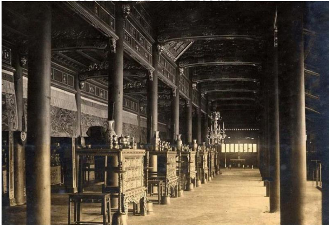
Figure 94: The historical interior photo of “The To Mieu” temple (1925)
