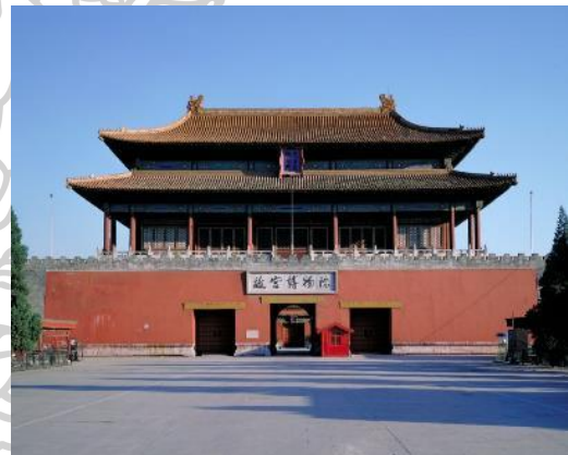
j) North gate (position 2)
