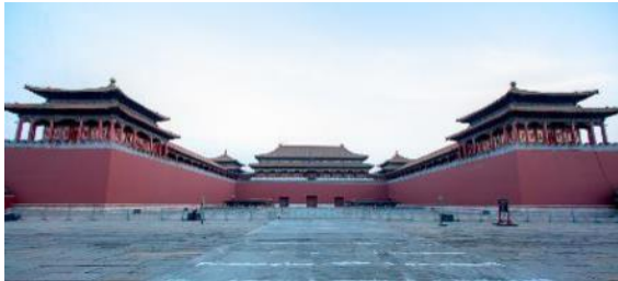
Figure 149a) Southern main gate (Figure 147, position 1) (Source: https://smarthistory.org/the-forbidden-city/ )
