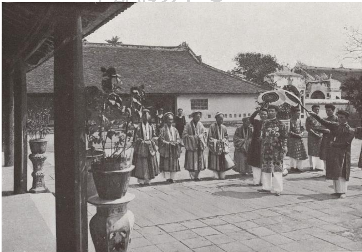
Figure 139: The historical photo of "Ta Tra Gia" house, viewed from "Dien Tho Chanh Dien" palace (1920-1925)
