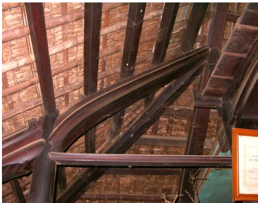
Figure 59: Using bamboo as a roof-structure for thatched roofing (Early Type C) (Source: Author)
