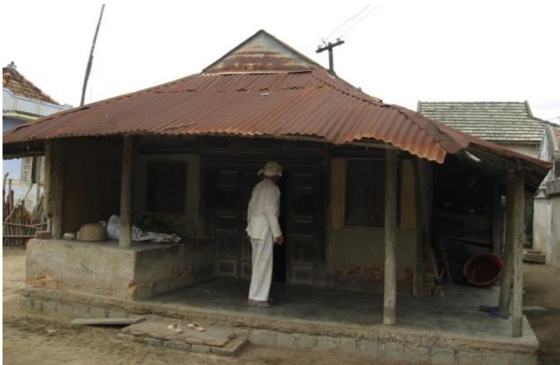
Figure 37: Front view of the “Nha Roi” (Early Type B), entrance in the direction of gable, house of Mr. Nai Nha, Phuoc Huu village, Phuoc Hau commune, Ninh Phuoc district, Ninh Thuan province (see Table 1, no. 59). (Source: Author)
