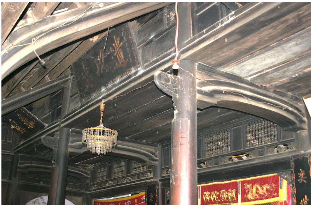
Figure 54: Wooden structure of the “Nha Ruong” (Later Type C), case of Mr. Le Hoi’s house, Hue City, Thua Thien Hue province (see Table 1, no. 17). (Source: An Khang company)
