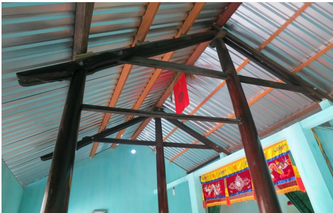
Figure 39: The reused-wooden frame of the “Nha Roi” (Early Type B) in Vietnamese’s house (Source: Author)
