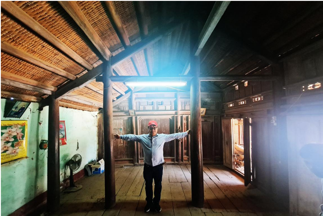
Figure 43:: The truss of the “Nha Roi” (Later Type B), entrance in the direction across the top-ridge beam, house of Mr. Quang Dai Hoang (Source: Author)
