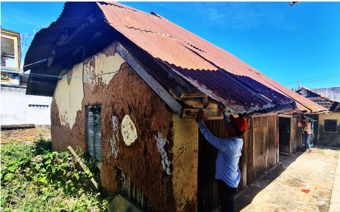
Figure 44:: The double roofed layers of the later Type B, above mentioned house of Mr. Quang Dai Hoang's family. (Source: Author)
