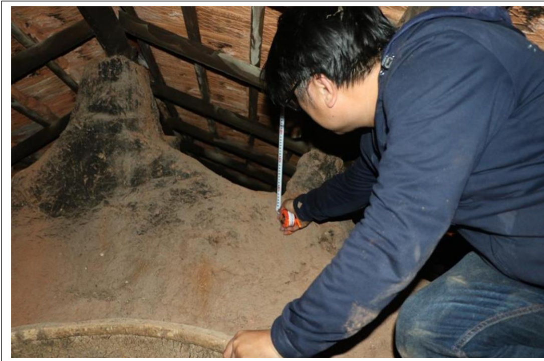
Figure AIII. 2.3 Survey clayed roof of Dương Thị Hương' house, Ly Hai commune, Ly Son island, Quang Ngai Province, (Source: Author ( 2021)
