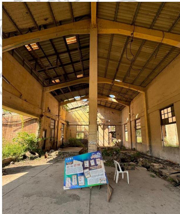
Figure 26: Structural elements and interior of Building C
