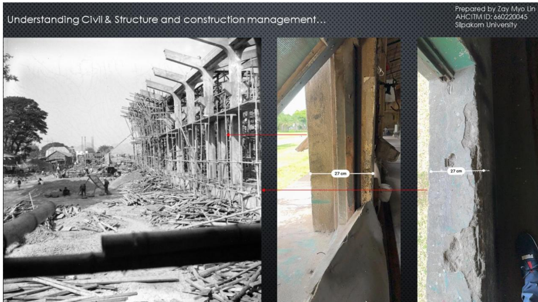
Figure 11: Walling work in progress in 1937 and onsite measurement conduct in 2024
