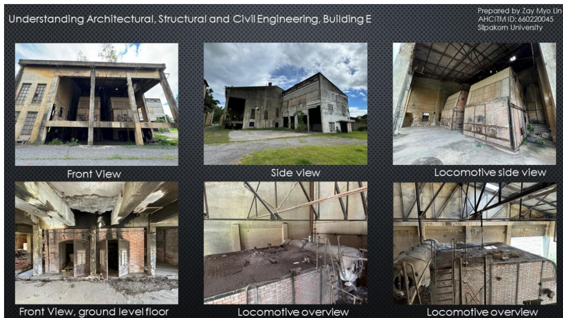
Figure 29: Architectural and overview of Building E, locomotive area
