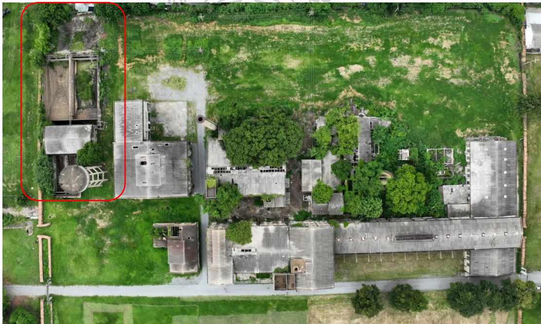
Figure 27: Building D group
