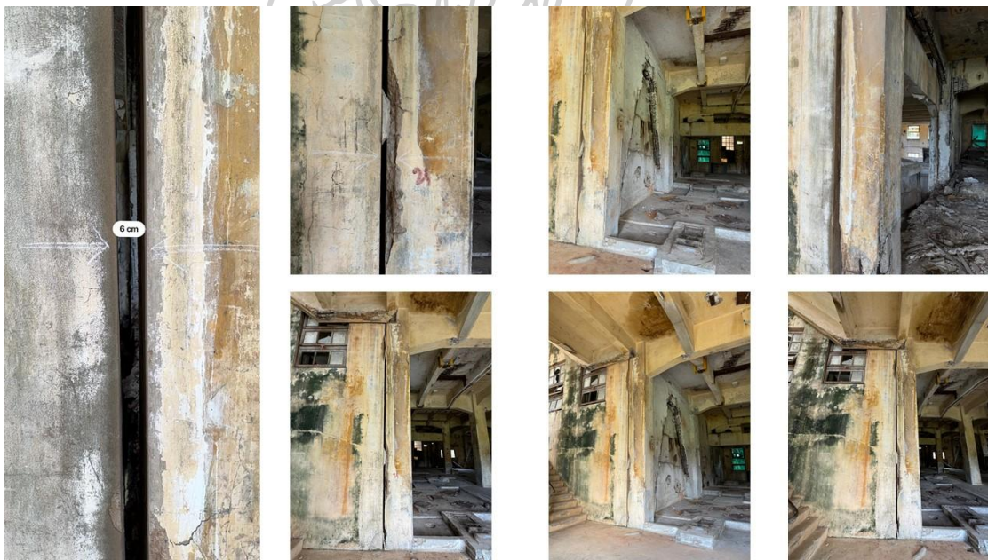
Figure 16: The two separate walls through bricklaying, which accounts for the existence of two separate walls
