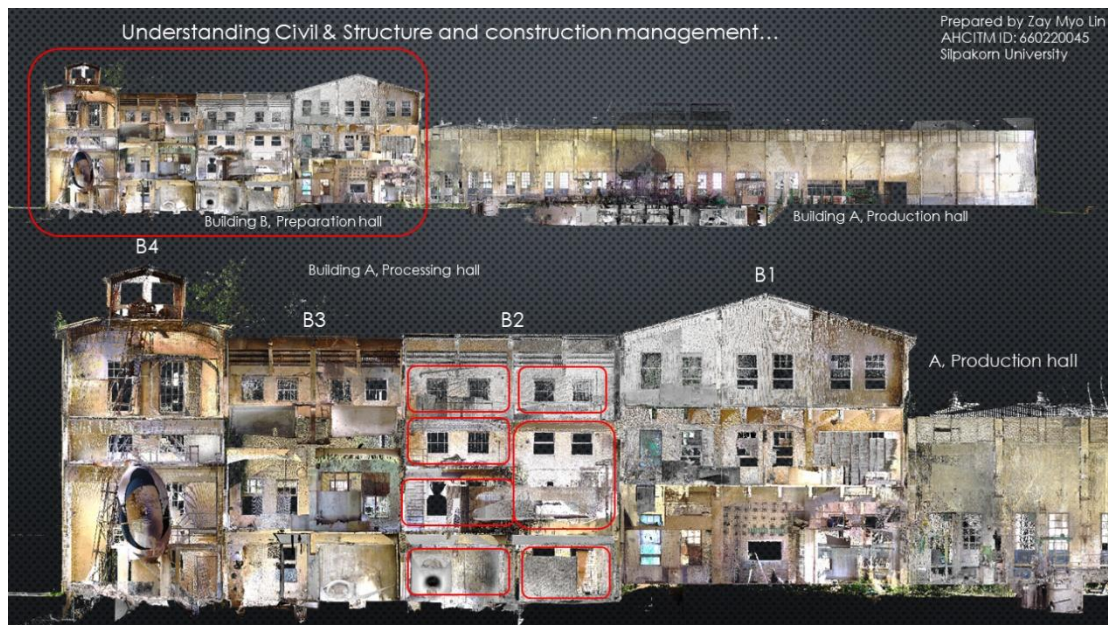
Figure 15: Section of Building B consist of 4 building 3D scanning by professor Isarachai Buranaut.
