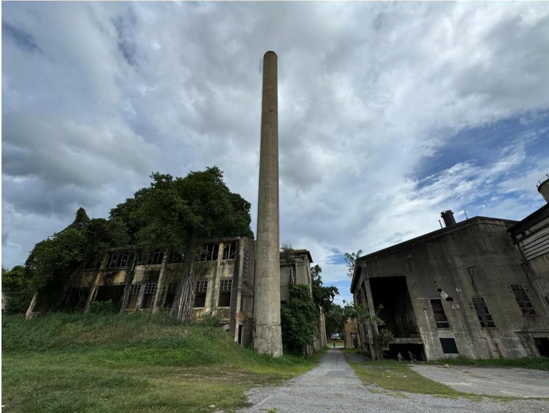
Figure 36: Reinforced concrete Industrial Chimney build in 1937 Photo by Zay Myo Lin (2024).
