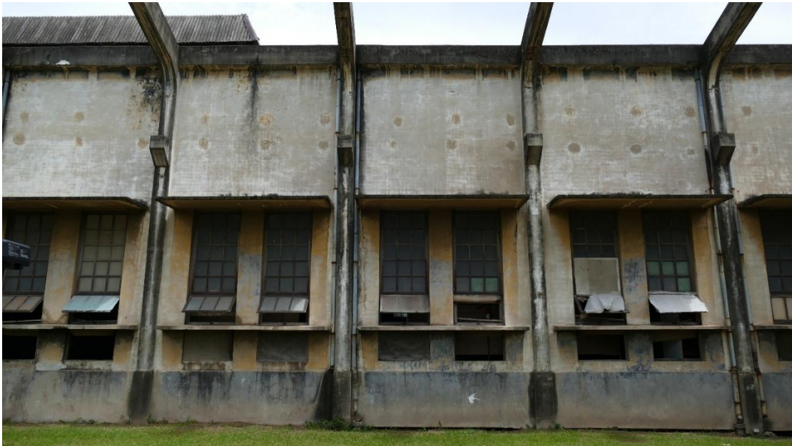
Figure 12: Façade and Window of Building A, Production Hall
