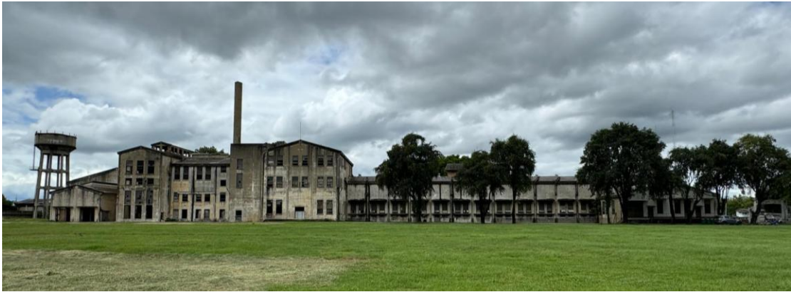
Figure 3: South side of Kanchanaburi paper mill
