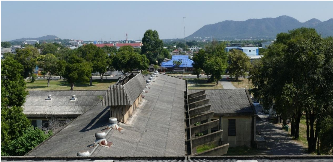
Figure 13: Roofing of Building A, Production Hall
