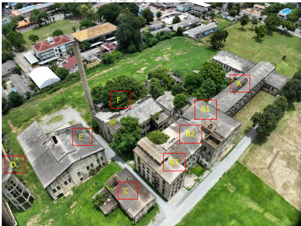
Figure 6: Existing Master Plan of Kanchanaburi Paper Mill complex. Aerial photo by Professor Isarachai Buranaut, 2024.
