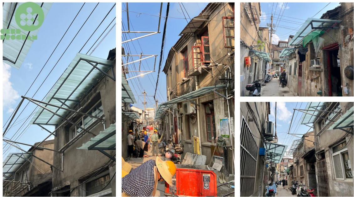
Figure 70 Actual effect after installation (Li, 2025)
