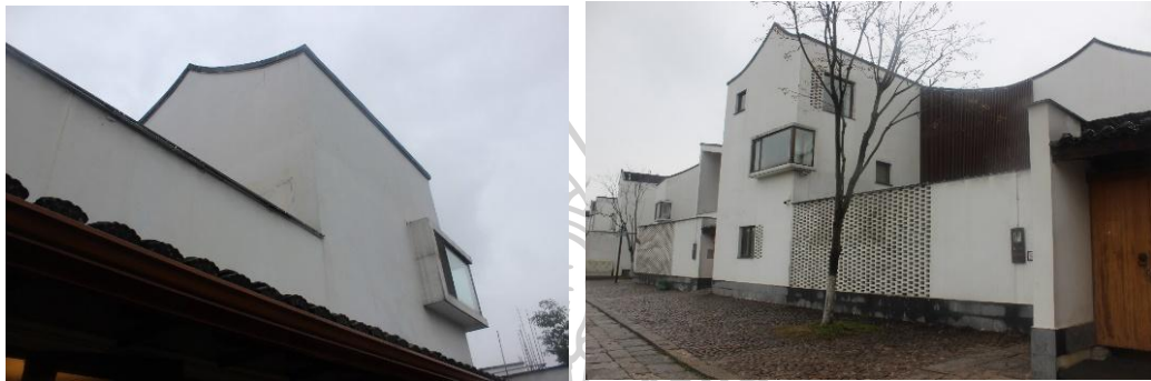
Figure 33 The roof of Dongziguan Village after the updated design (Li, 2022)
