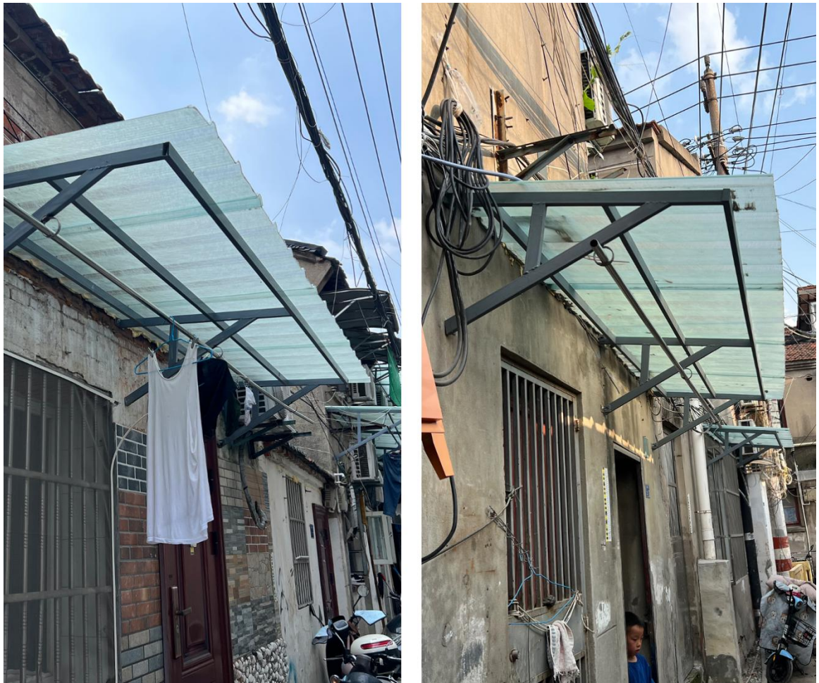
Figure 72 Actual effect after installation (Li, 2025)
