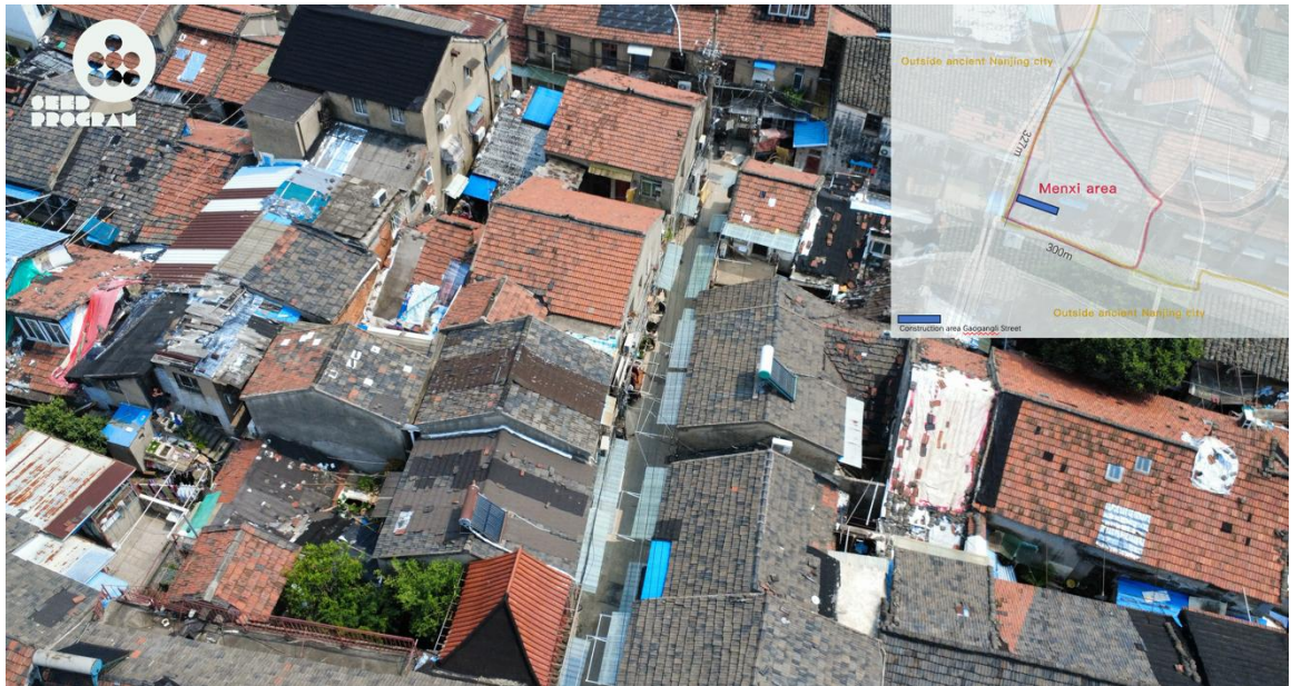
Figure 71 Actual effect after installation (Li, 2025)
