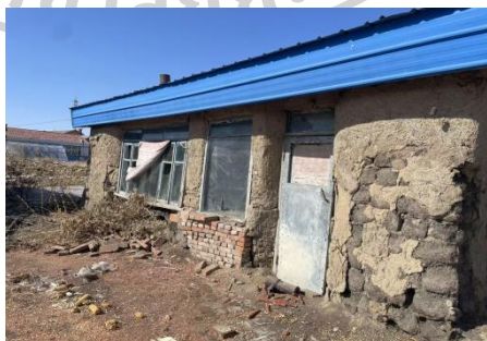
Figure 102 Wooden beams + iron sheets: approximately 18%
