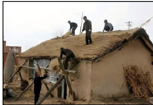
Figure 75 Thatched roof laying
