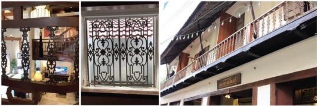
Figure 24 Ornamentation at balcony
