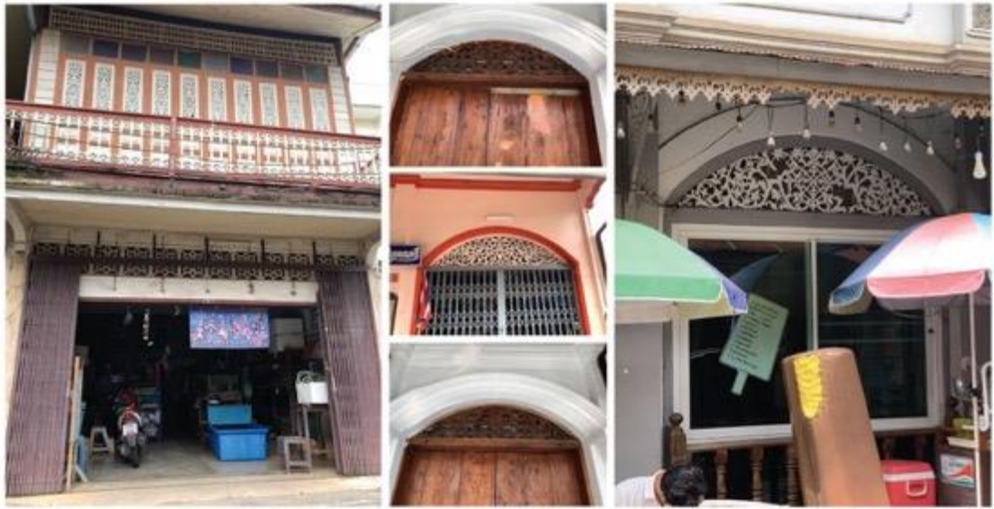
Figure 21 Ornamentation above doors area
