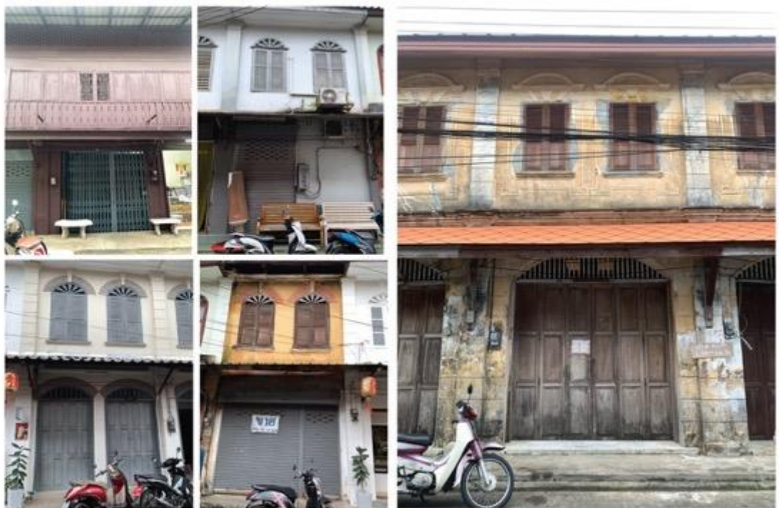
Figure 22 Ornementation under beams Source: Kanlayanee Phueaknamphol, 2023
