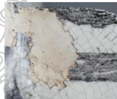
Figure 29 : Close-up of area exhibiting lifting, loss of glaze layer.
