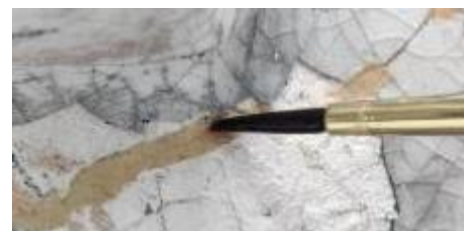
Figure 47 : Close-up of the application of protective coating.
