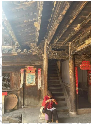
Figure 23 The Wooden Beam-Column Framework
