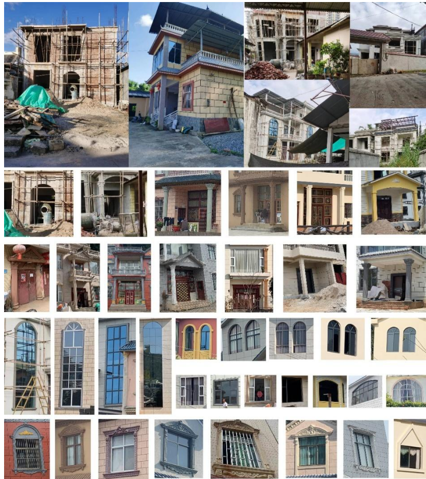
Figure 40 European-Style Dwellings and Architectural Details in the Third Wave of Rural Construction
