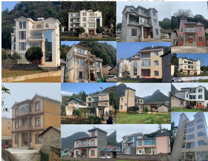
Figure 1 Contemporary Rural Dwellings in Central Yunnan
