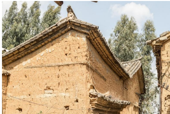
Figure 27 Bricks at the Eaves
