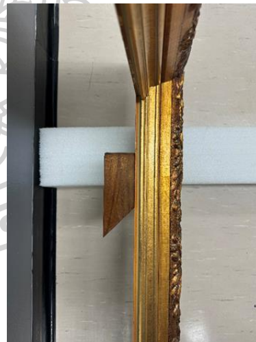
Figure 39: French cleat-like hanging system.
