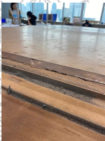
Figure 44: Dirt and dust accumulated on auxiliary support.
