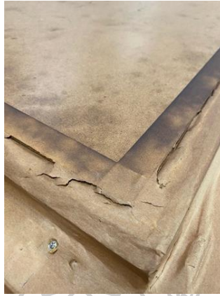
Figure 42: Darkened water-activated paper tape.
