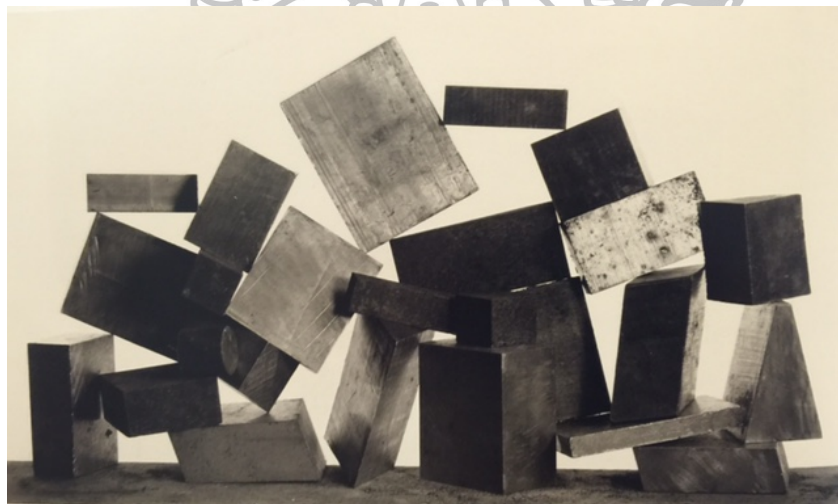
Figure 44 Collapse, New York 1990
