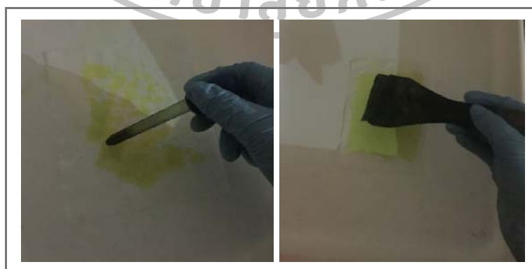
Figure 66 Using dropper to drop the chemical on the surface. Spreading the chemical with Hake brush
