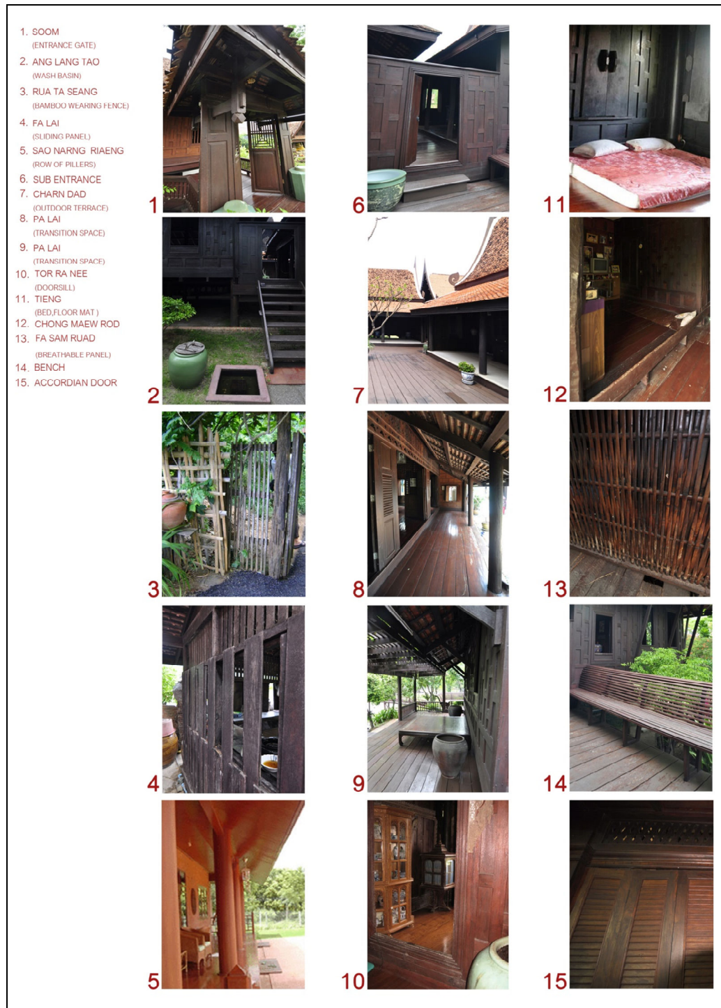
Figure 76 Identical Elements of Thai House, The above table shows the tangibly essential elements of Thai house that concluded by researcher, all 15 elements could be generally founded in Thailand.
