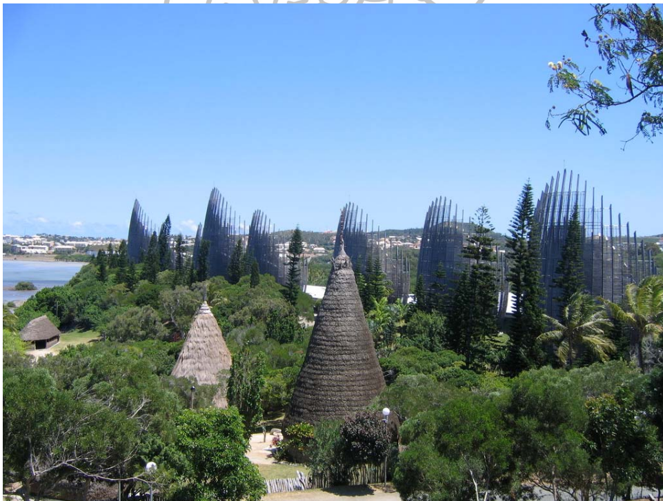
Figure 43 The tradition architecture and new design alongside together
