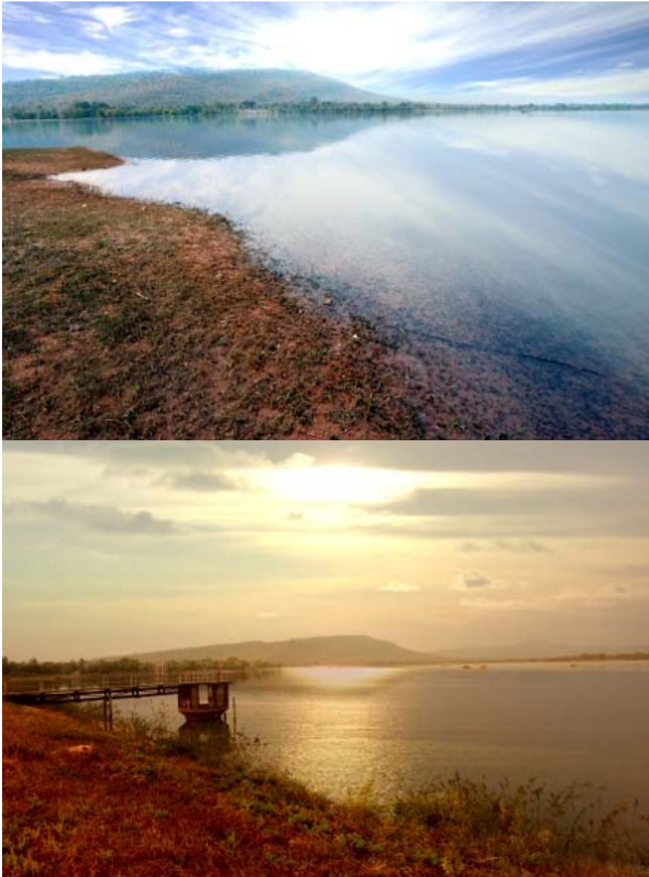
Figure 99 Huai Chumchang Dam.
