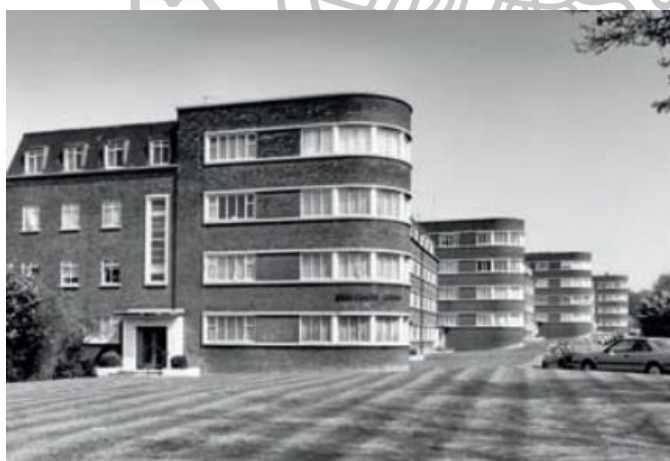
Figure 62 Belvedere Court flats, Lyttelton Road, designed by Ernst Freud in 1935, with bold 'streamform' bays. [Hampstead Garden Suburb Trust (Jane Whitton)]
