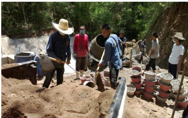
Figure 77 Check Dams Building (2)
