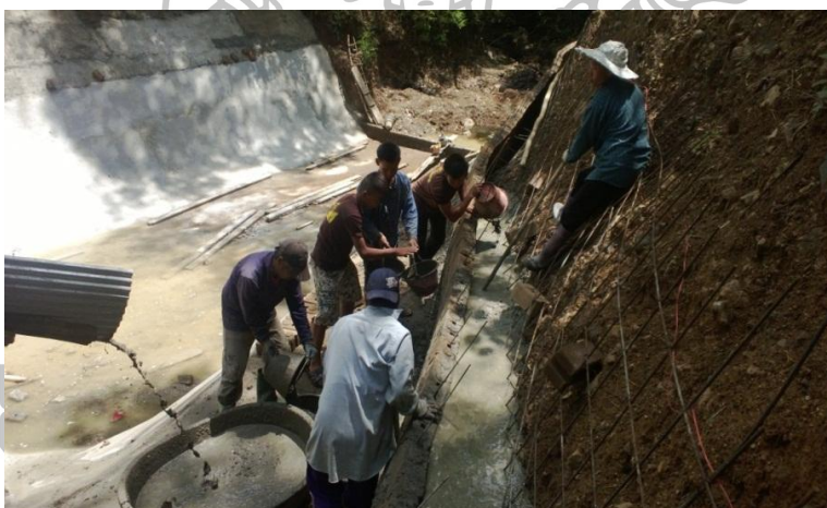
Figure 78 Check Dams Building (3)
