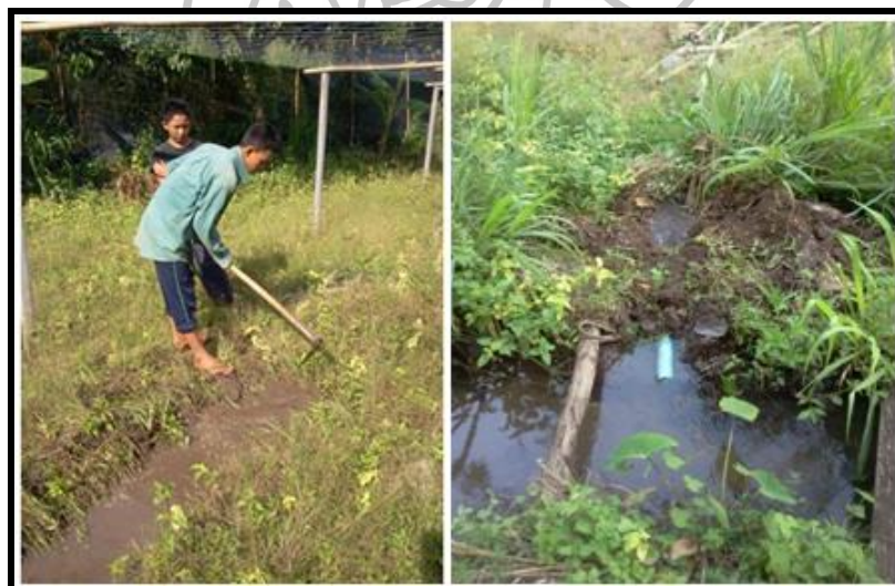
Figure 54 Dredging the water course
