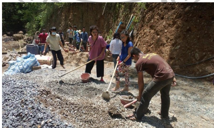
Figure 76 Check Dams Building (1)
